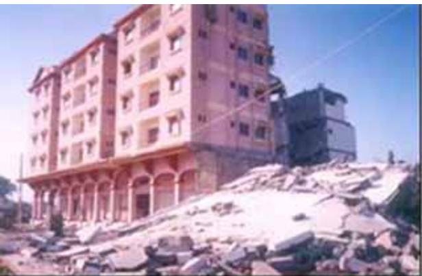
Fig. 19: Gujarat Earthquake, 2001 by UNCRD (India)
