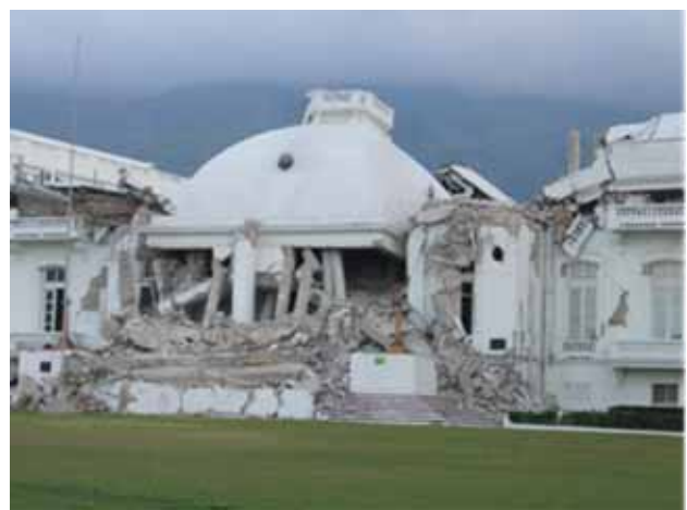
Fig. 16: Damage of President Office, 2010 by CODE (Haiti)
