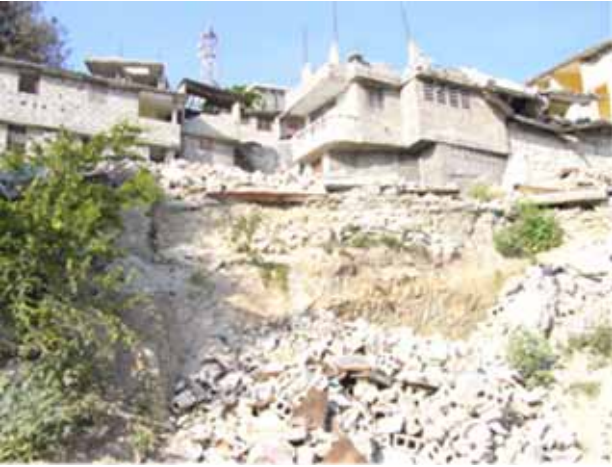
Fig. 17: Landslide in residential area, 2010 by CODE (Haiti)
