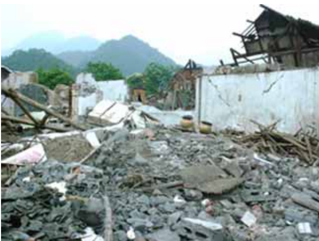
Fig. 12: Damaged wooden/brick houses, 2008 (Sichuan)
