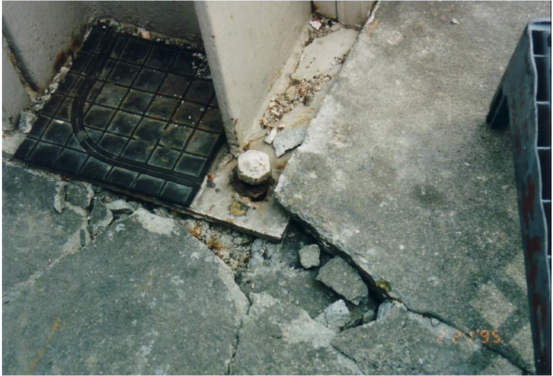
Photo 3.2.2-29 Minor damage on an exposed column base
