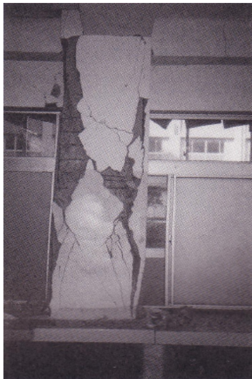
Photo 3.2.3-6 Concrete seriously came off to expose reinforcement to a large extent, but without buckling or deformation
