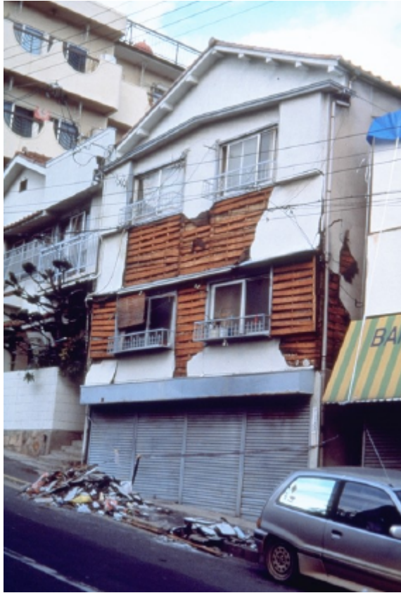
Photo 3.2.2-43 Damage on a wall (exterior wall) (Rank C)
