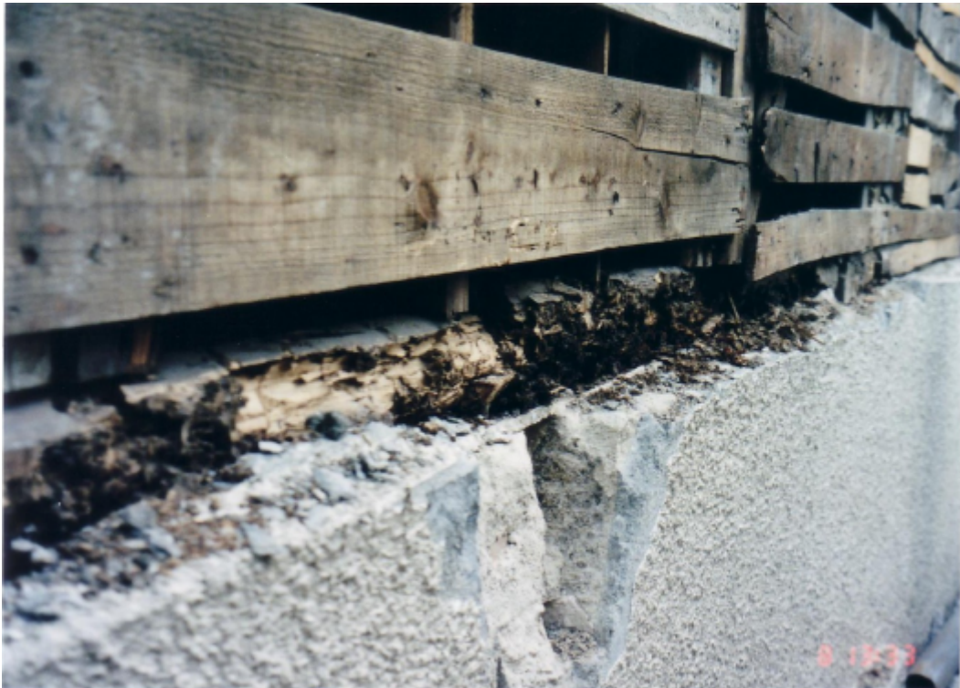
Photo 3.2.2-44 Ant damage (Rank C)
