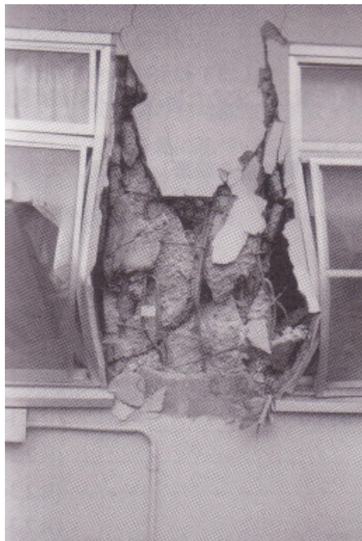
Photo 3.2.3-10 The main reinforcement buckled, hoop hock disconnected, and inside concrete that came off with apparent deformation into the vertical and horizontal directions.
