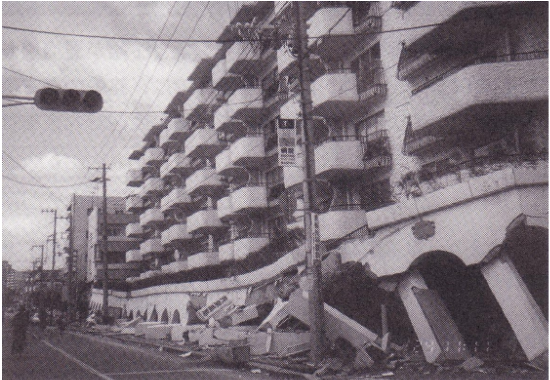
Photo 3.2.3-13 The 1st floor columns broken to cause a story collapse and the 2nd story and above fallen down.
