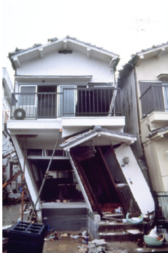
Photo 3.2.2-38 Tilting of a building at the first floor (Rank C)
