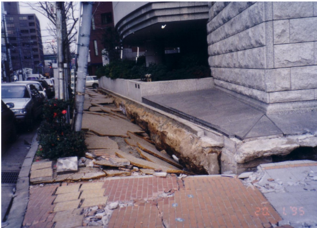
Photo 3.2.3-23 Surrounding area of the building settled due to ground liquefaction
