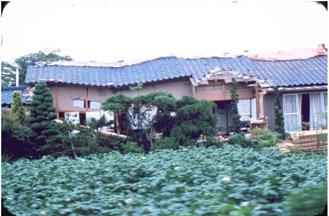
Photo 3.2.2-34 Differential settlement of a building (Rank B)
