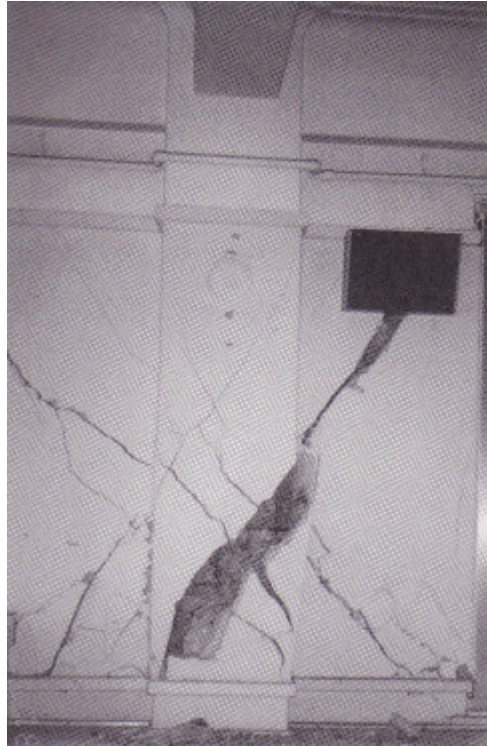
Photo 3.2.3-9 A number of large diagonal cracks on the wall and column to expose reinforcement without buckling, break, or deformation in the vertical direction.
