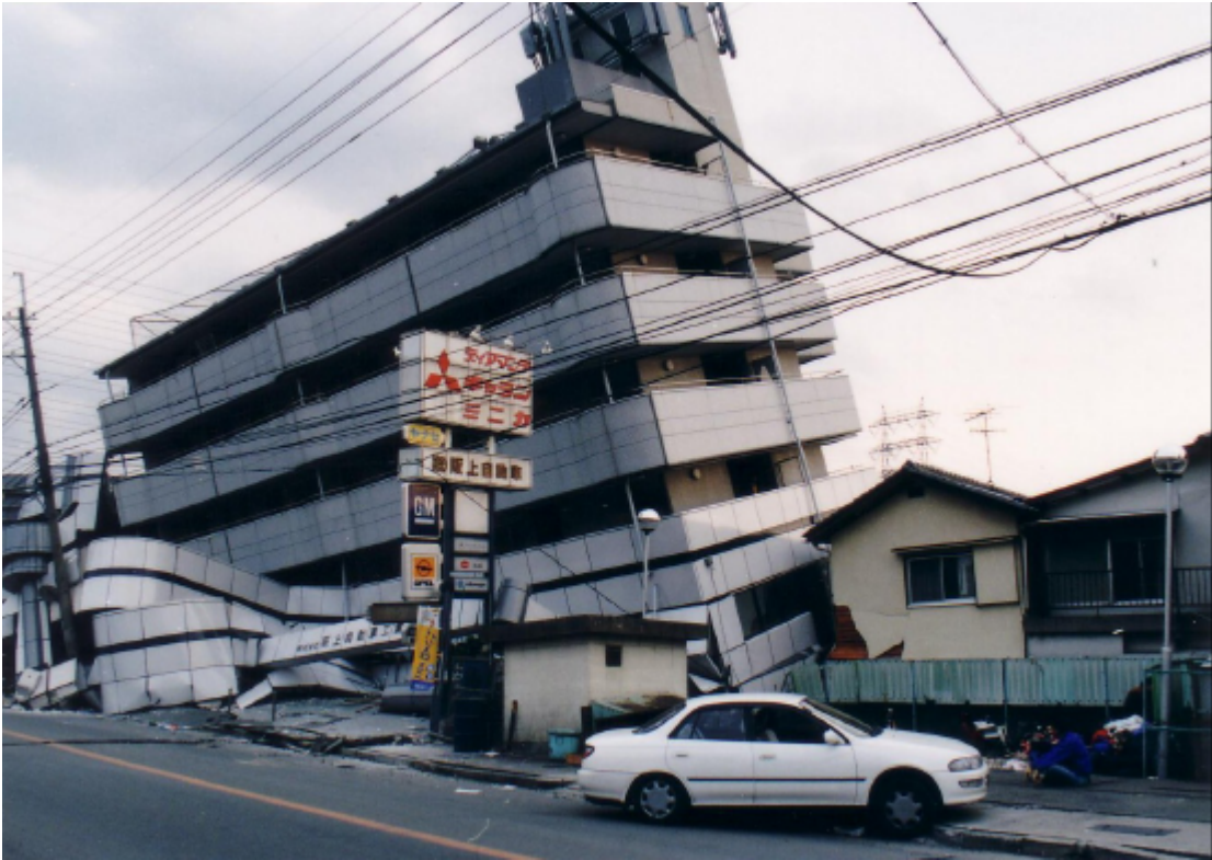
Photo 3.2.2-11 A building collapsed at low stories.
