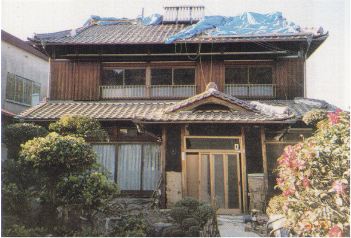
Photo 3.2.2-37 Tilting of a building at the first floor (Rank B)
