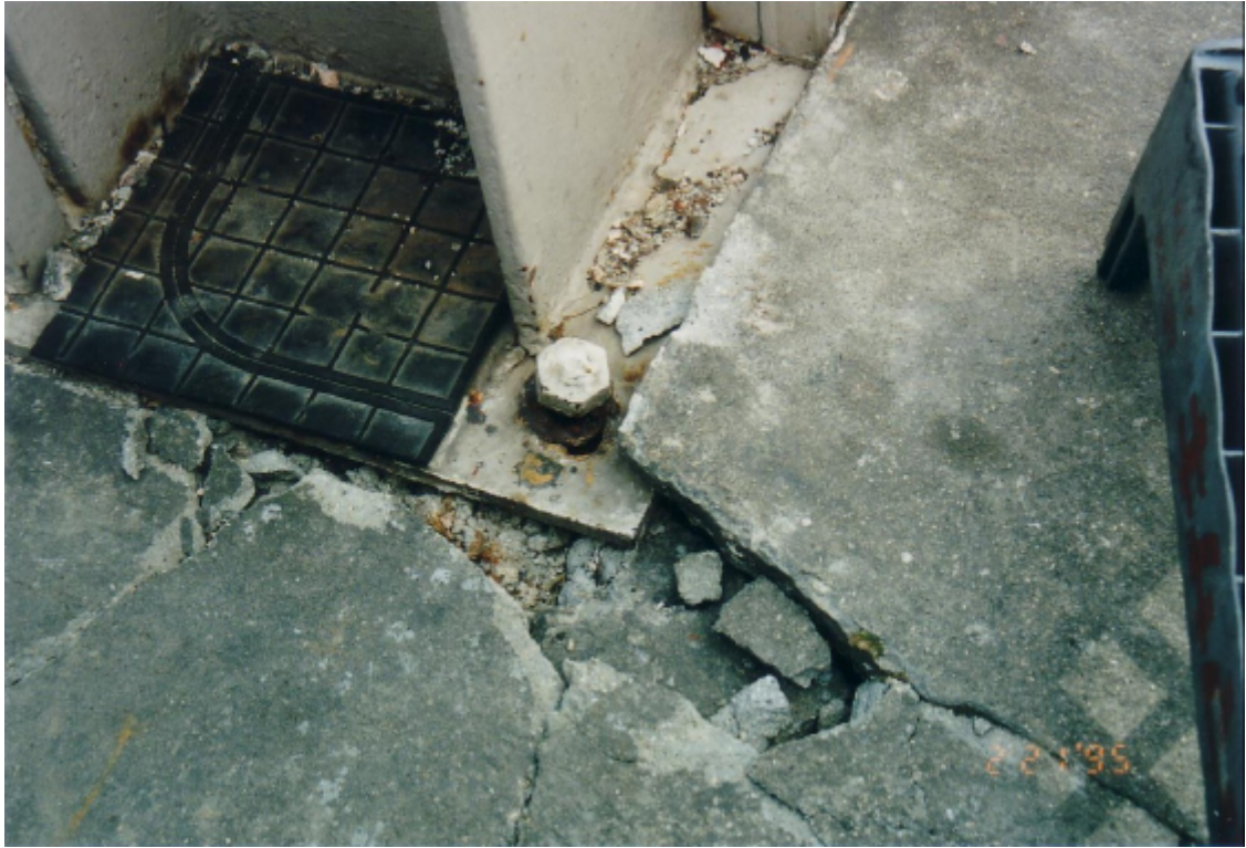
Photo 3.2.3-36 Minor damage on an exposed column base
