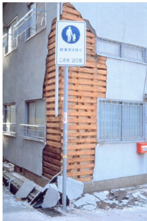
Photo 3.2.2-42 Damage on a wall (exterior wall) (Rank B)
