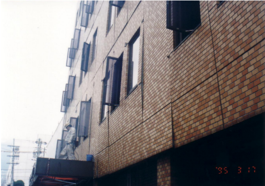
Photo 3.2.3-16 Damage of the PC curtain wall of a 5-story, moment resisting frame structure office building
