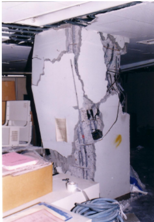
(b) The column capital and base have fractured due to bending shear and have deformed the column in the vertical direction.
