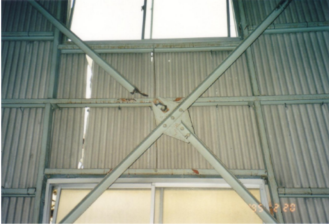
Photo 3.2.3-30 Rupture of angle braces
