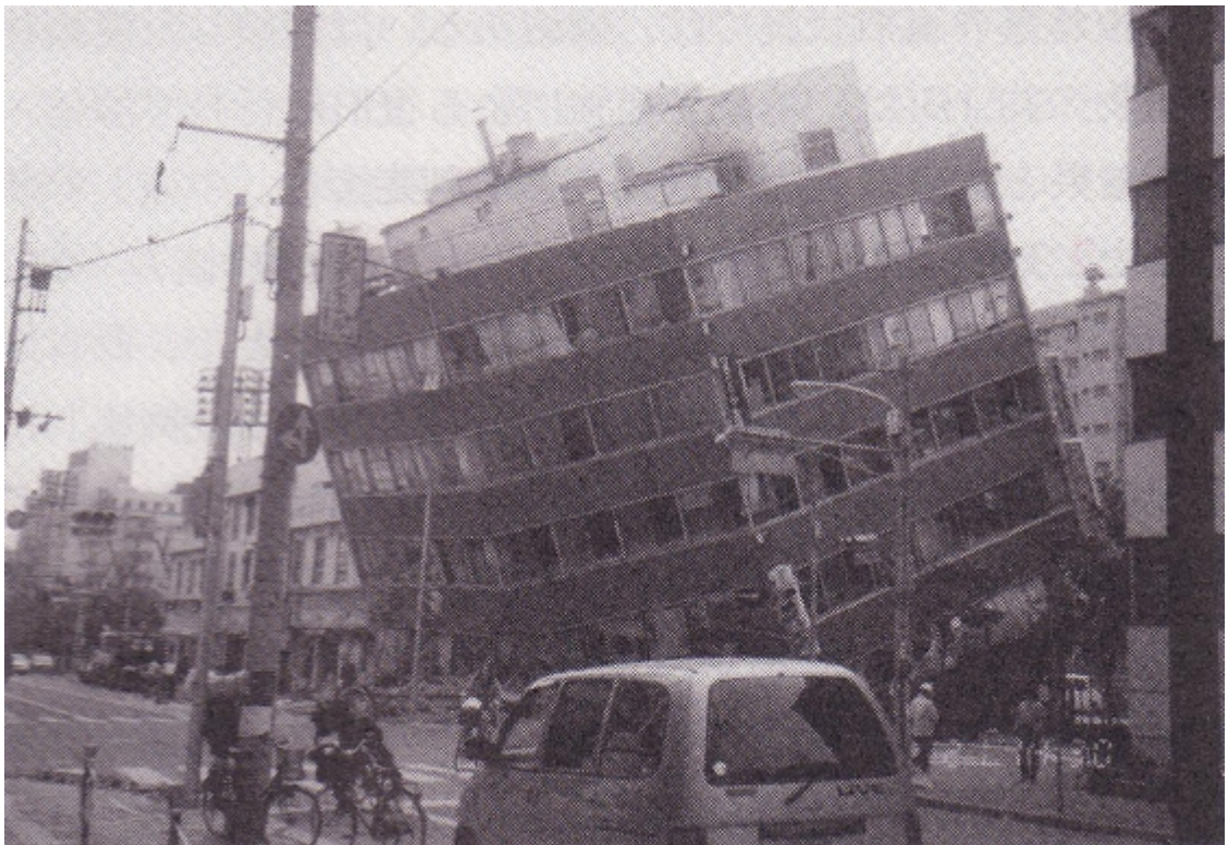
.Photo 3.2.3-14 The 1st floor columns broke thus significantly tilting the entire building
