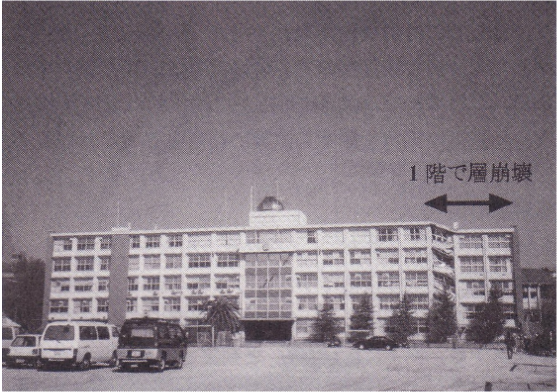
Photo 3.2.3-15 The three spans of the 1st floor on the right side have broken and caused a story collapse. On such a building, the damage should be judged separately for the three spans and the rest of the building.
