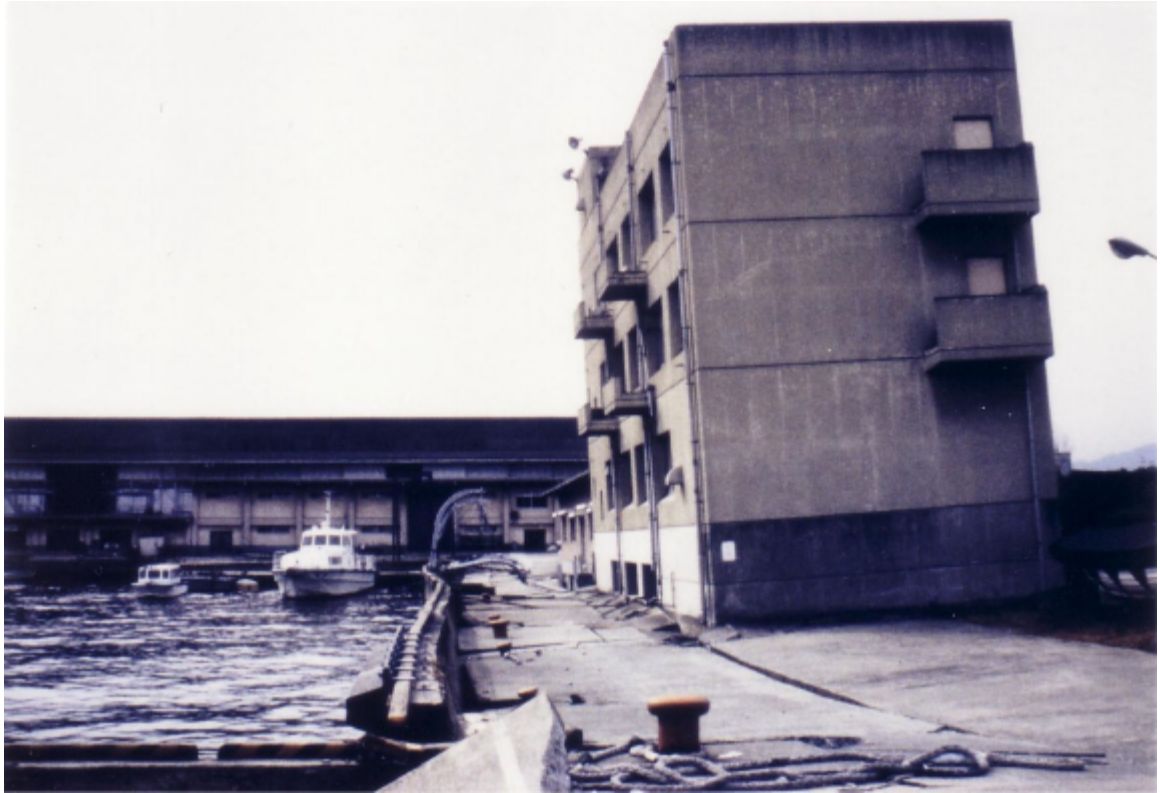
Photo 3.2.2-17 A building inclined due to the lateral flow of the ground (displacement of bulkhead)
