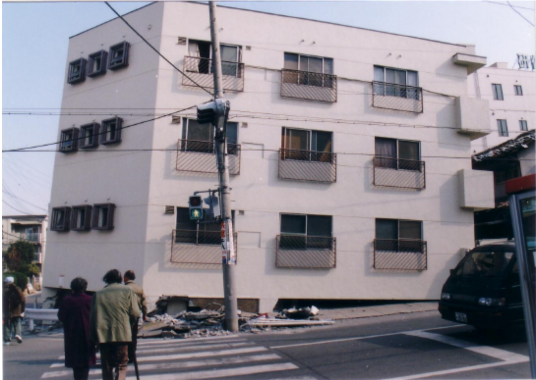
Photo 3.2.2-5 Example of building tilting at 2 degrees or more
