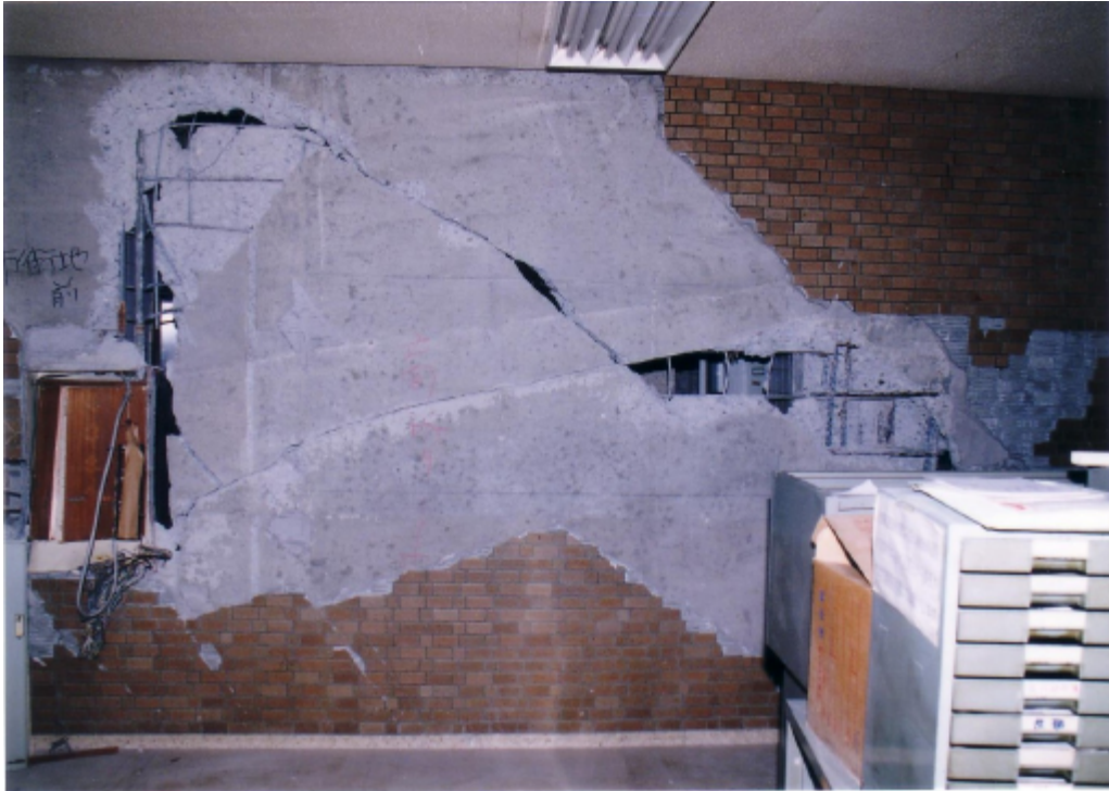
(c) See-through shear cracks on a wall; also the wall and column reinforcement bars are significantly bent.
