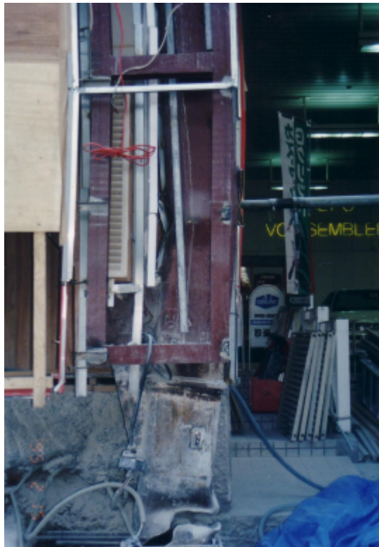
Photo 3.2.2-22 A totally buckled column
