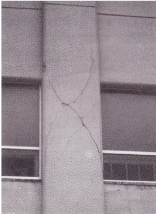
Photo 3.2.3-1 About 2-mm-wide X-shaped cracks on the column and large cracks on the covering concrete
