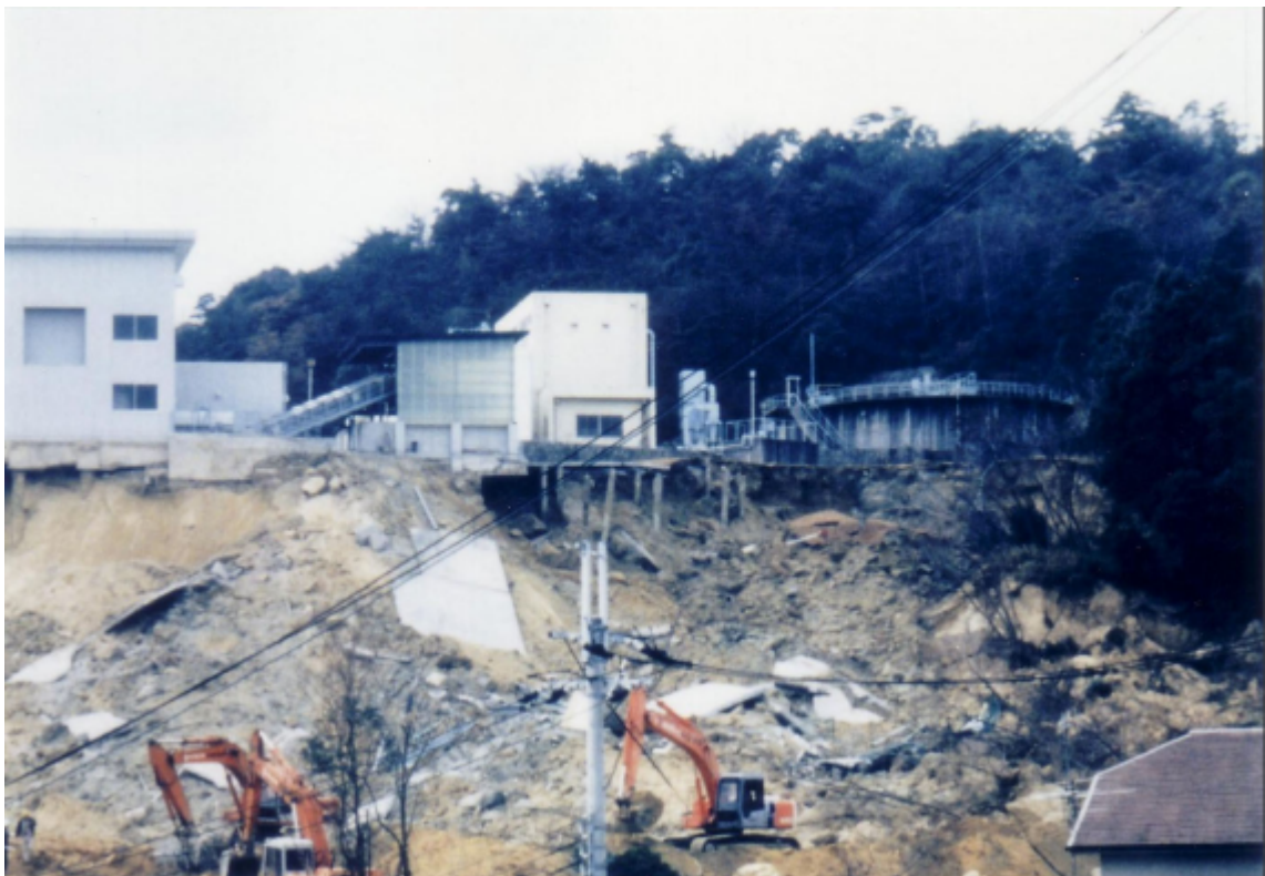
Photo 3.2.2-14 Danger of building site collapse
