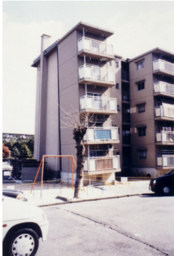
Photo 3.2.2-18 A condominium inclined due to differential settlement
