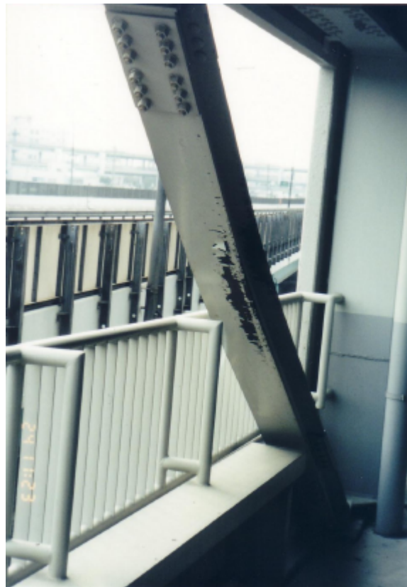
Photo 3.2.3-31 Buckling of wide-flange-shaped braces
