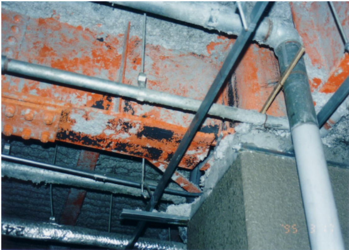
Photo 3.2.2-10 Yield and fracture of a beam end inside a 5-story, moment resisting frame structure office building
