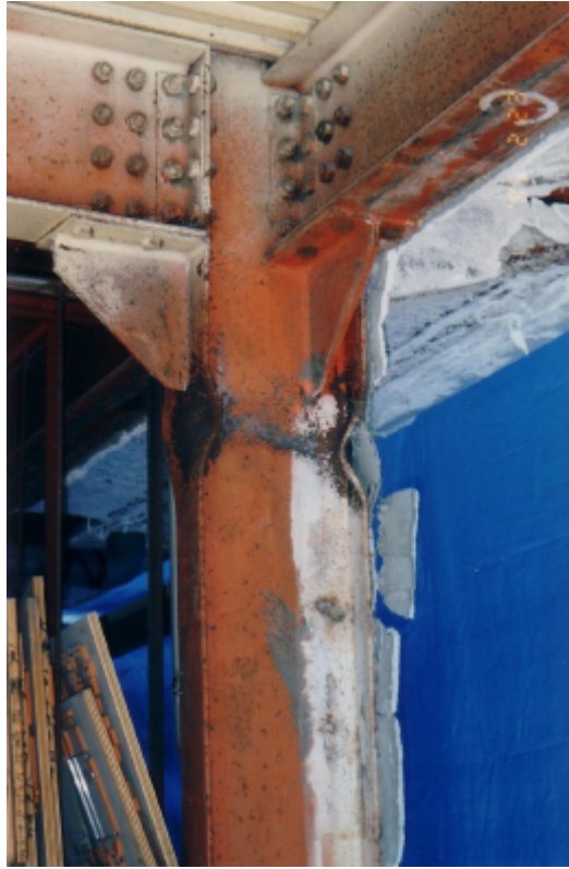
Photo 3.2.2-21 A locally buckled column
