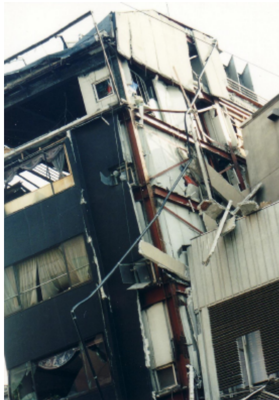
Photo 3.2.2-12 A building inclined to a large extent
