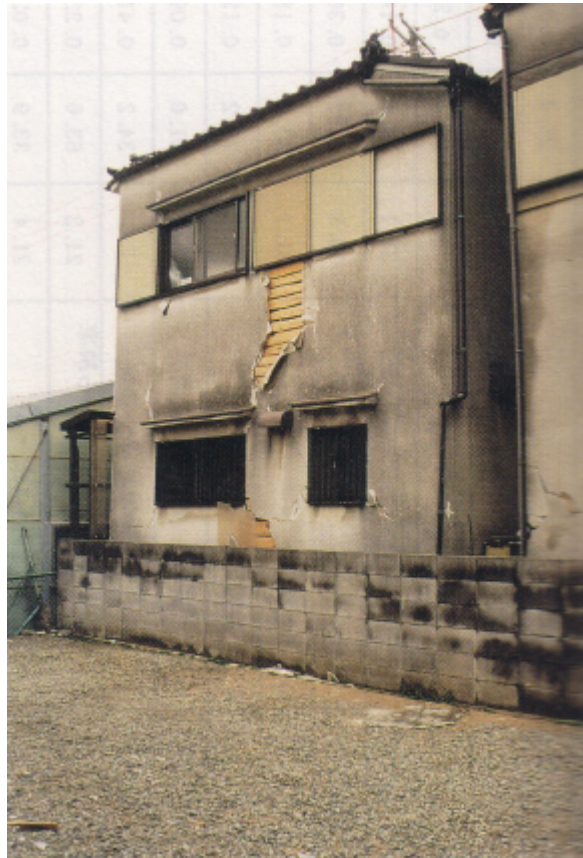
Photo 3.2.2-41 Damage on a wall (exterior wall) (Rank B)
