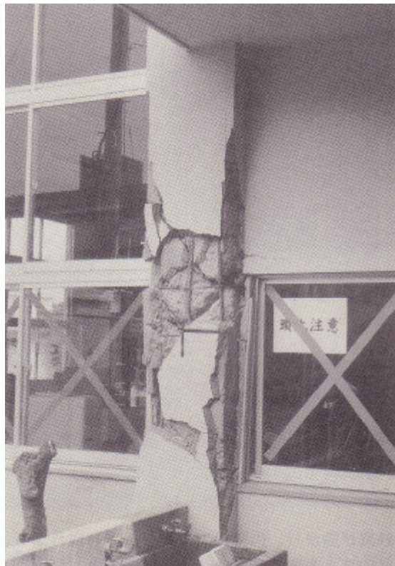
(c) A large volume of concrete has come off and has exposed reinforcement bars in a wide area. If the column has deformed in the vertical direction, the damage will be at the level V.
