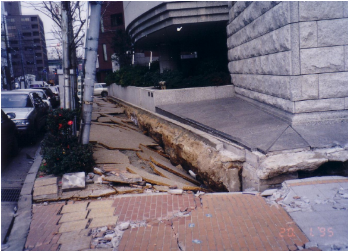
Photo 3.2.2-16 Surrounding area of the building settled due to ground liquefaction
