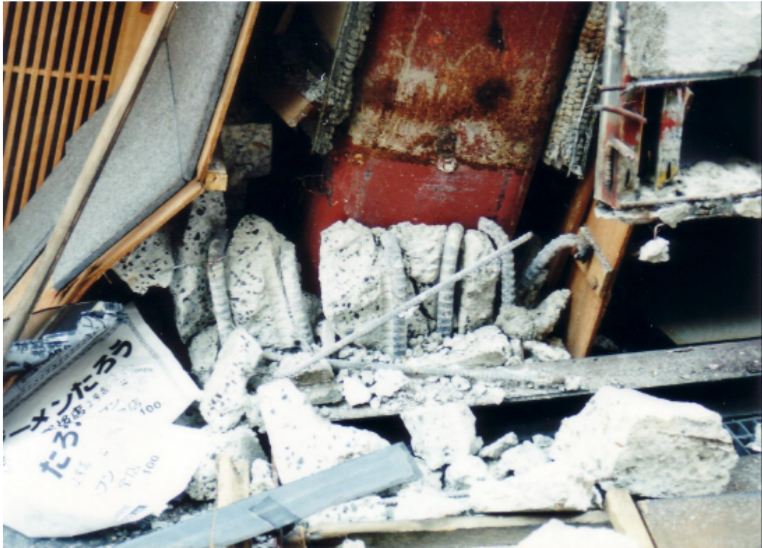
Photo 3.2.2-27 Displacement of a concrete column base of insufficient encasing height
