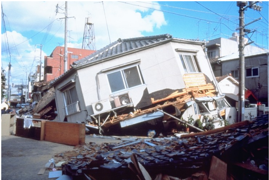
Photo 3.2.2-32 A scene of apparent unsafe
