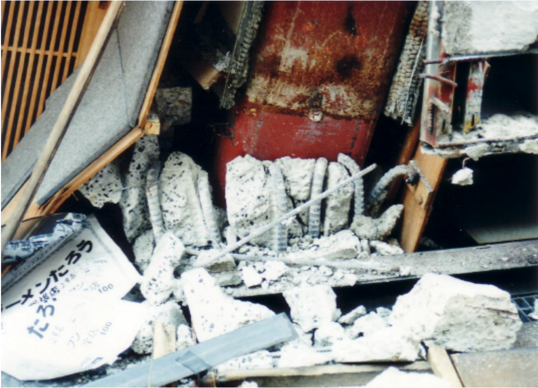
Photo 3.2.3-34 Displacement of a concrete column base of insufficient encasing height
