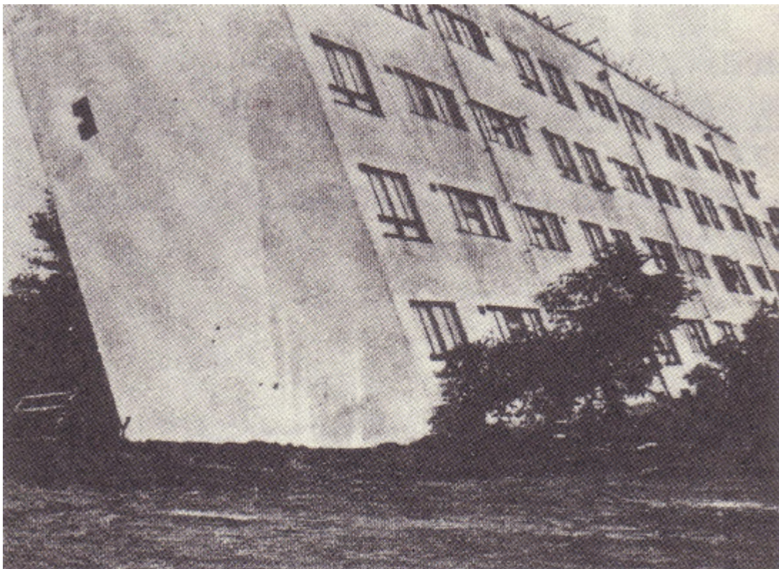
Photo 3.2.2-4 Example of the sinking and tilt of an entire building.
