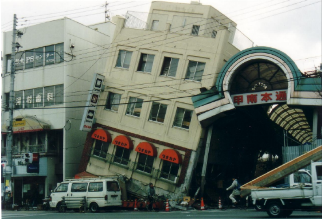
Photo 3.2.2-15 A building with the risk of collapse
