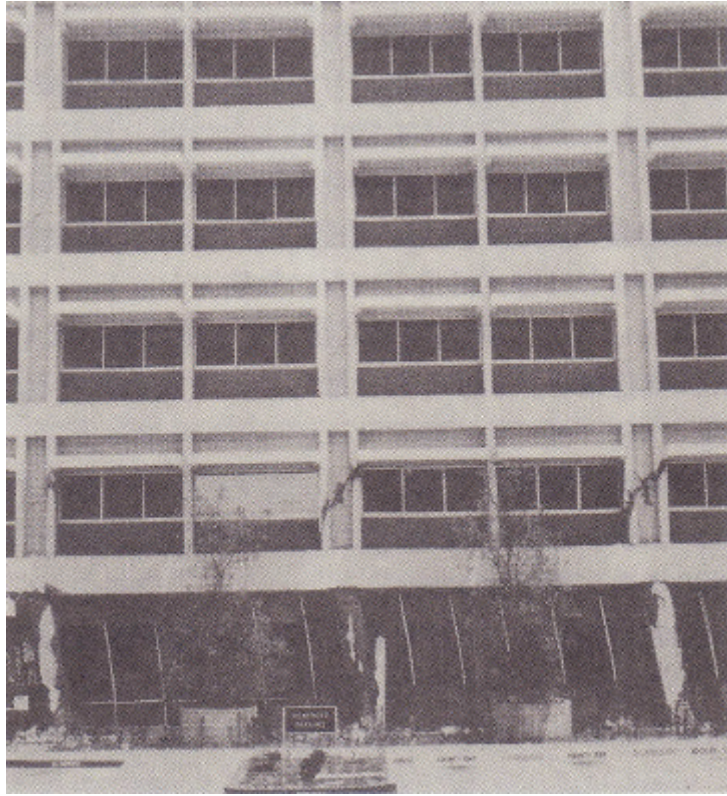
Example of the damage due to a large horizontal deformation caused by the damage of columns
