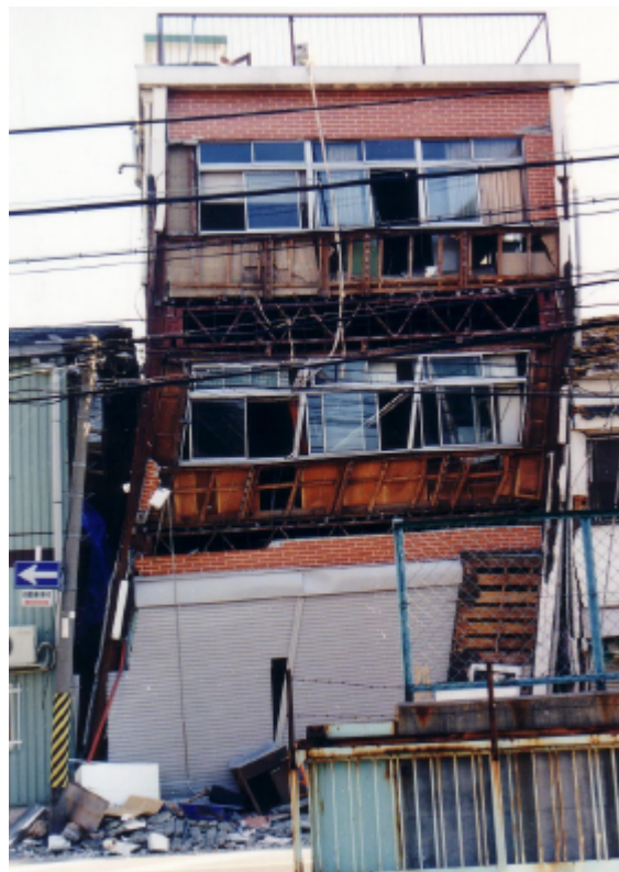
Photo 3.2.2-20 A building inclined at the 1st and 2nd floors only
