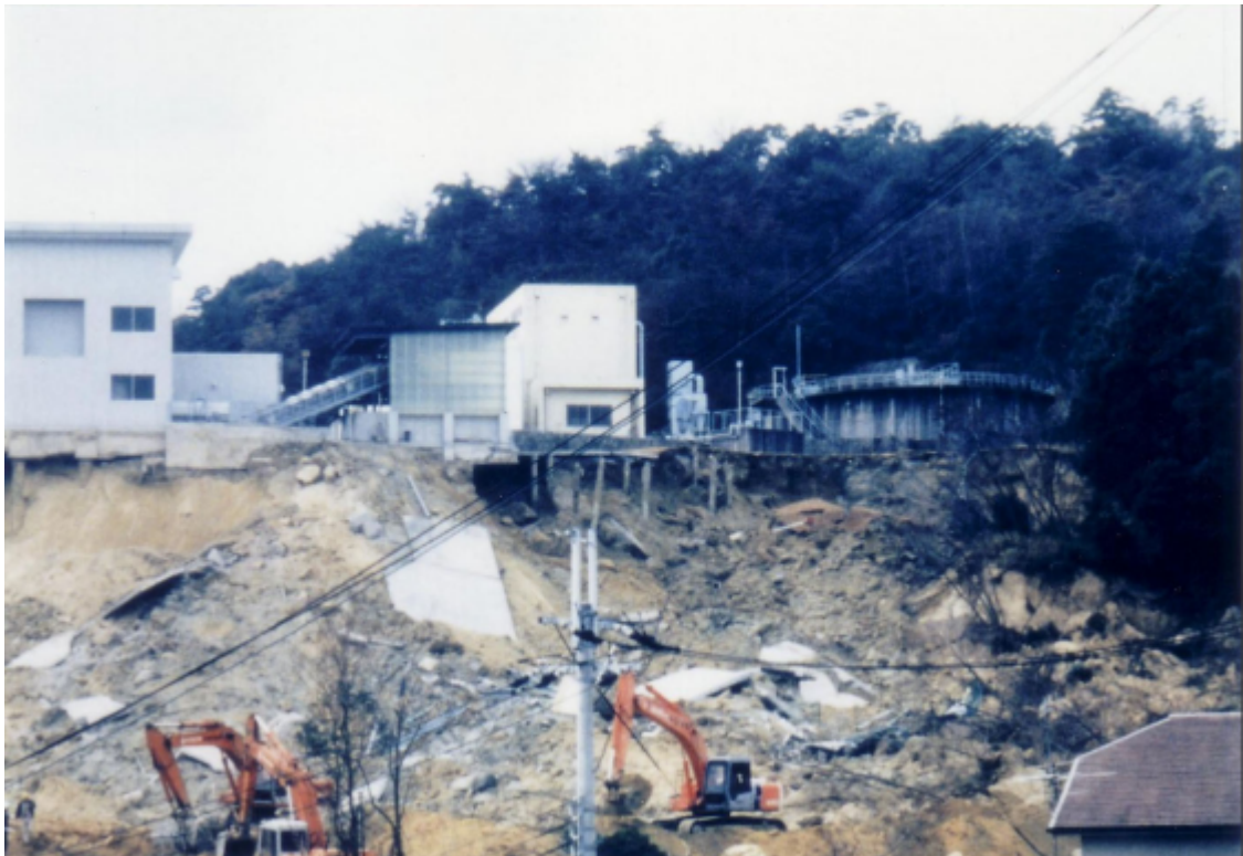
Photo 3.2.3-21 Danger of building site collapse
