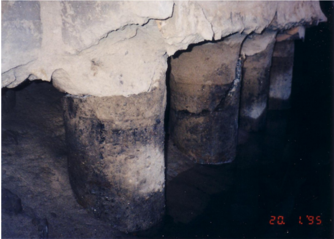
Photo 3.2.2-13 Serious damage of piles
