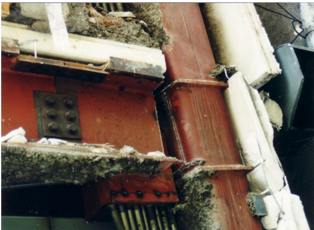
Photo 3.2.2-25 Rupture of a welded beam end
