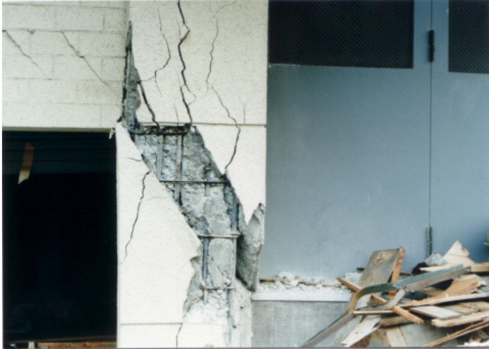
(b) A large volume of concrete has come off and has exposed reinforcement bars in a wide area.
