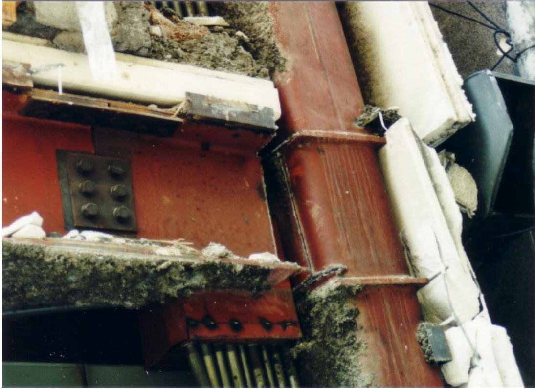
Photo 3.2.3-32 Rupture of a welded beam end
