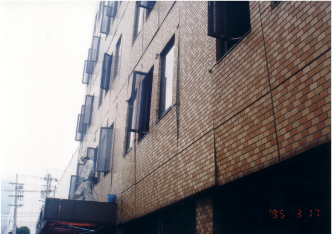
Photo 3.2.2-9 Damage of the PC curtain wall of a 5-story, moment resisting frame structure office building
