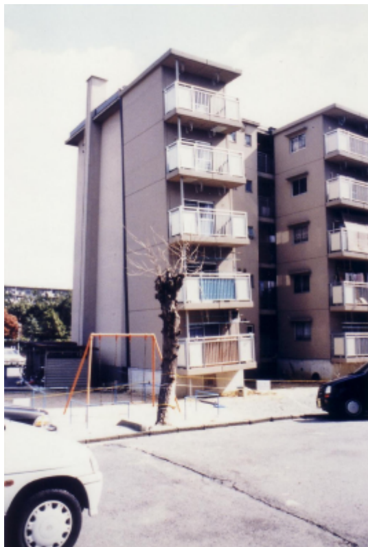
Photo 3.2.3-25 A condominium inclined due to differential settlement
