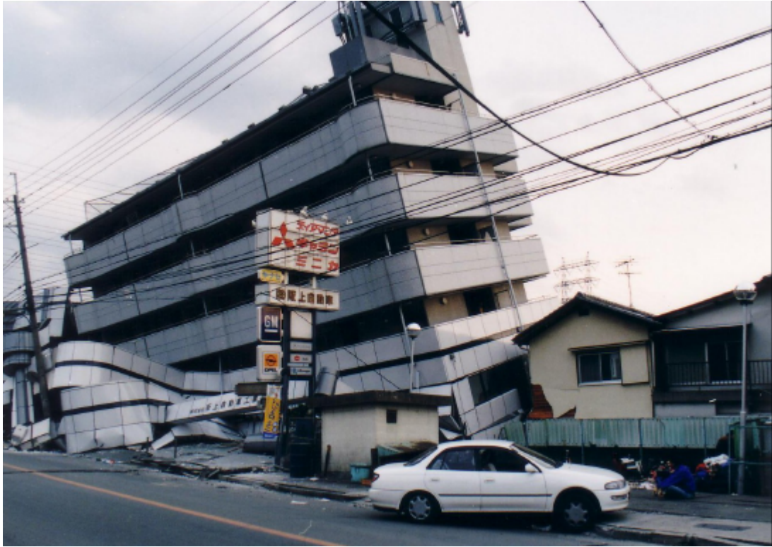
Photo 3.2.3-18 A building collapsed at low stories.
