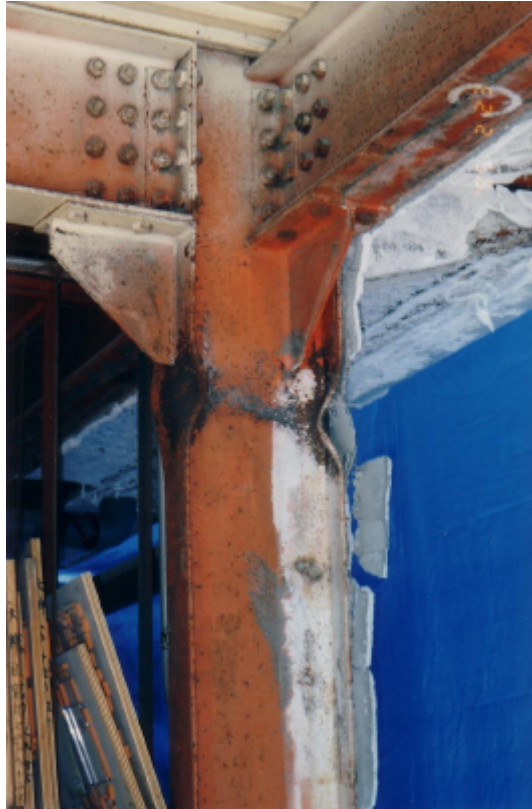
Photo 3.2.3-28 A locally buckled column
