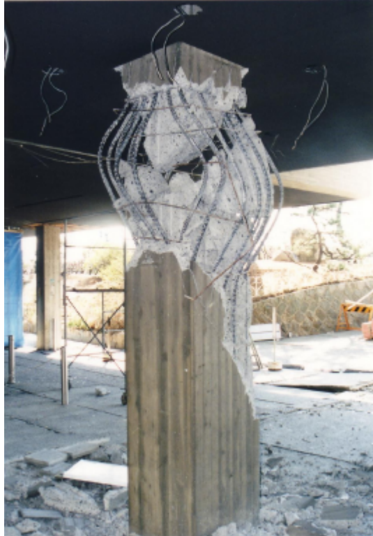
(a) The reinforcement bars have bent and the concrete inside the column has collapsed. The column has deformed in the vertical direction.
