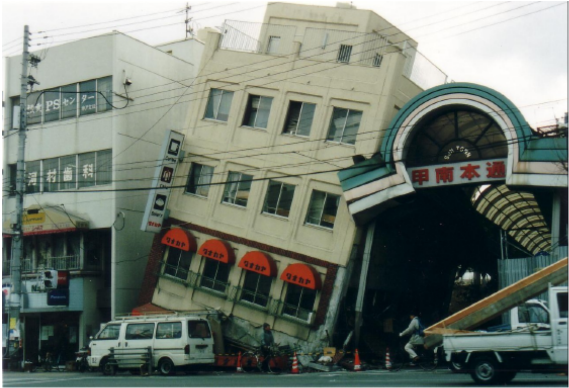
Photo 3.2.3-22 A building with the risk of collapse
