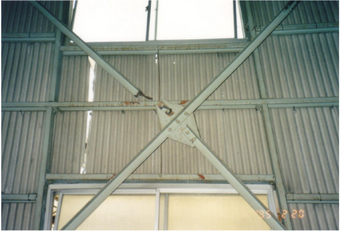
Photo 3.2.2-23 Rupture of angle braces
