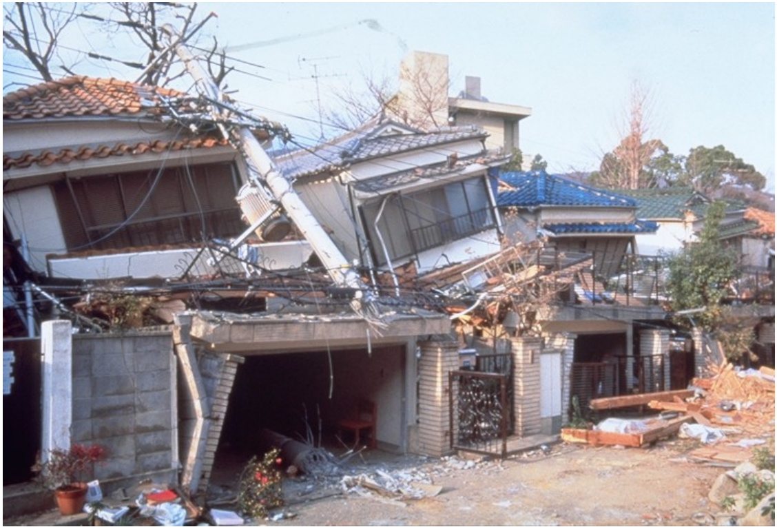
Photo 3.2.2-31 A scene of apparent unsafe
