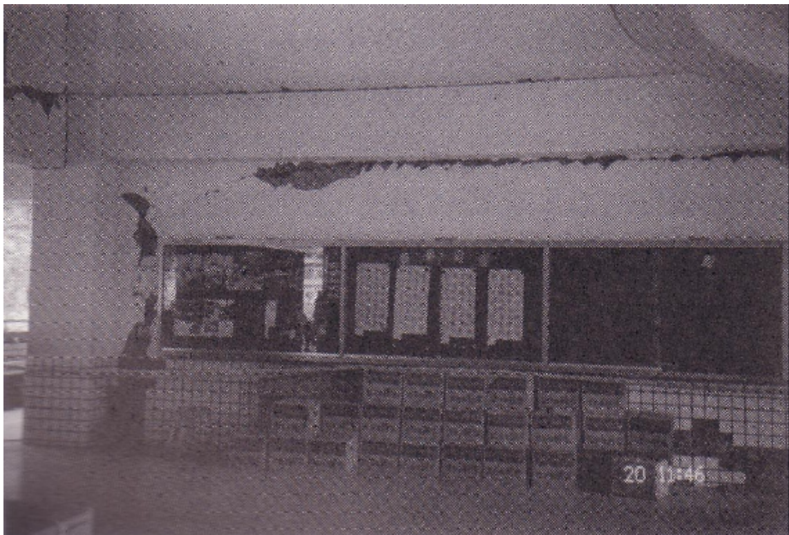
Photo 3.2.3-4 Diagonal cracks on the wall and cracks at the joint between lower beam part and wall plate that is caused by sliding without deformation of vertical wall reinforcement.
