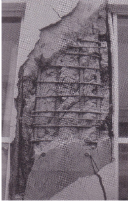
Photo 3.2.3-5 Cracks wider than 2 mm on the column with concrete that came off to expose reinforcement, but without buckling or deformation
