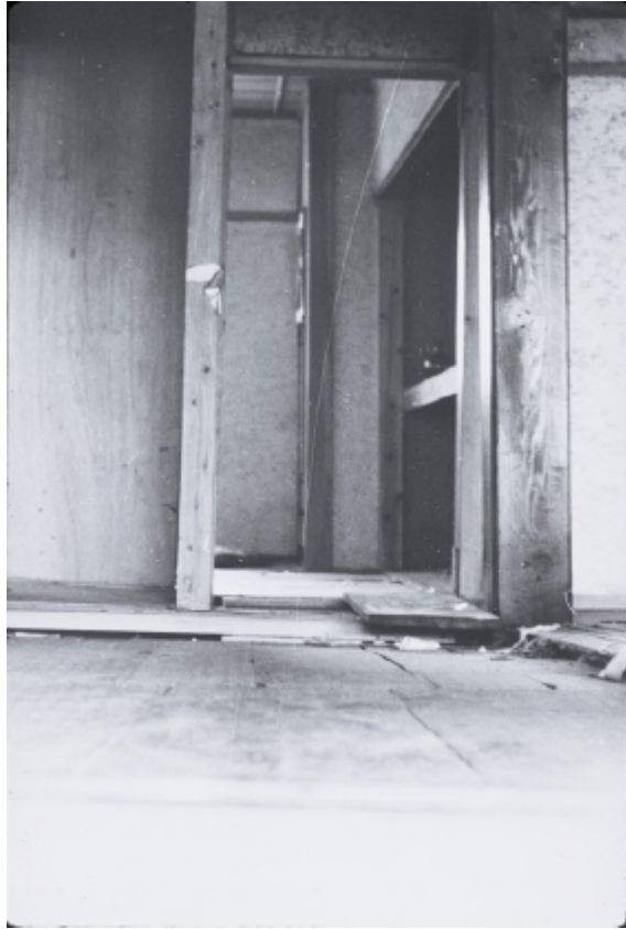
Photo 3.2.2-33 Differential settlement of a building (Rank A)
