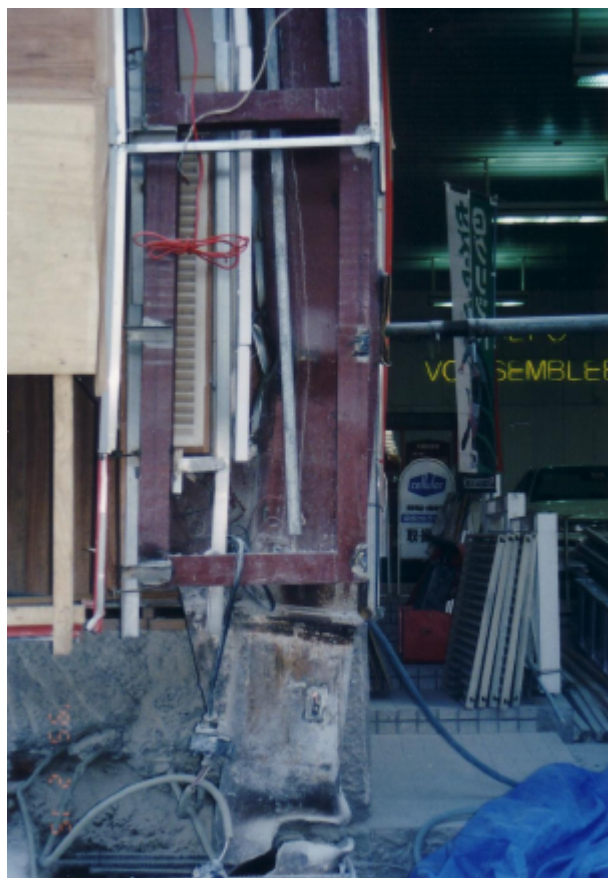
Photo 3.2.3-29 A totally buckled column
