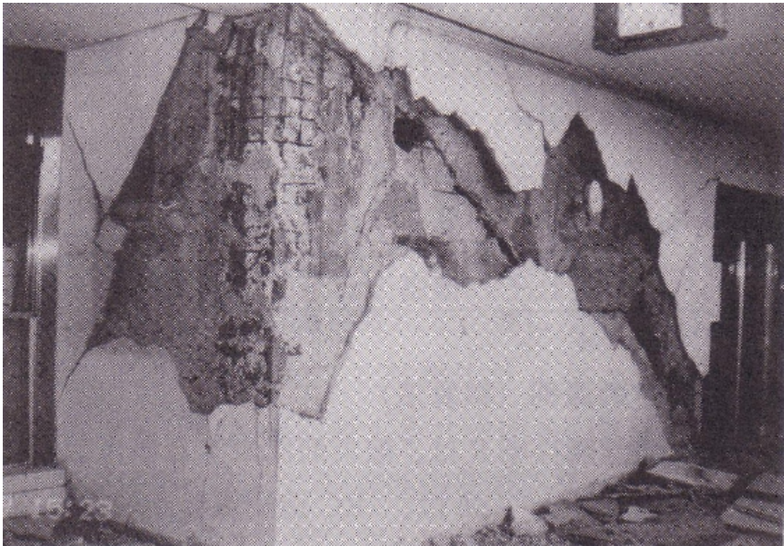
Photo 3.2.3-12 Large and oblique see-through diagonal cracks on the wall with concrete coming off.
