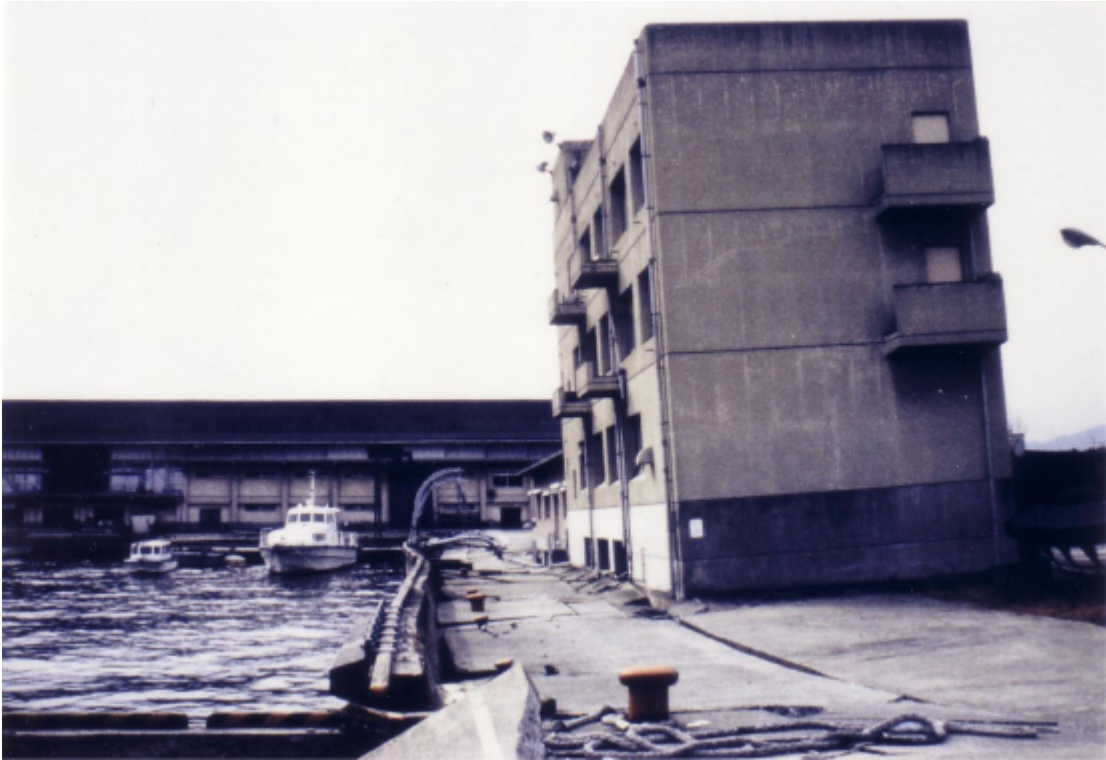
Photo 3.2.3-24 A building inclined due to the lateral flow of the ground (displacement of bulkhead)
