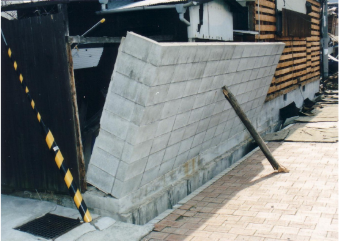
Photo 3.2.2-49 An object that can overturn (block wall) (Rank C)
