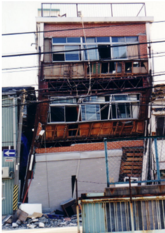
Photo 3.2.3-27 A building inclined at the 1st and 2nd floors only
