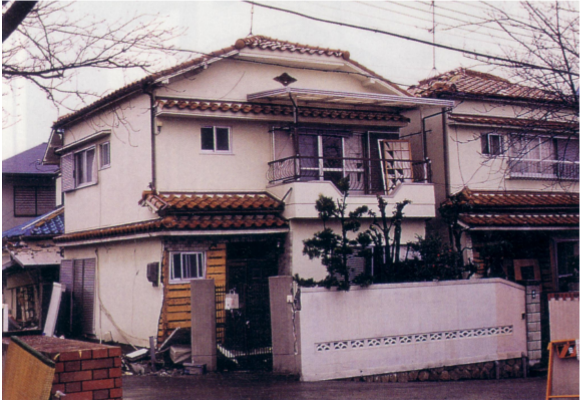
Photo 3.2.2-39 Damage on a wall (exterior wall) (Rank B)
