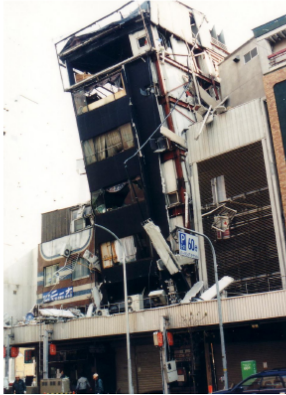
Photo 3.2.2-19 An inclined building
