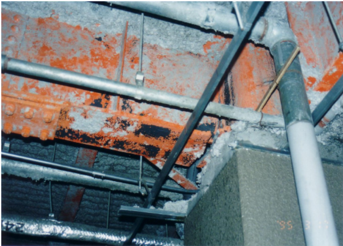
Photo 3.2.3-17 Yield and fracture of a beam end inside a 5-story, moment resisting frame structure office building
