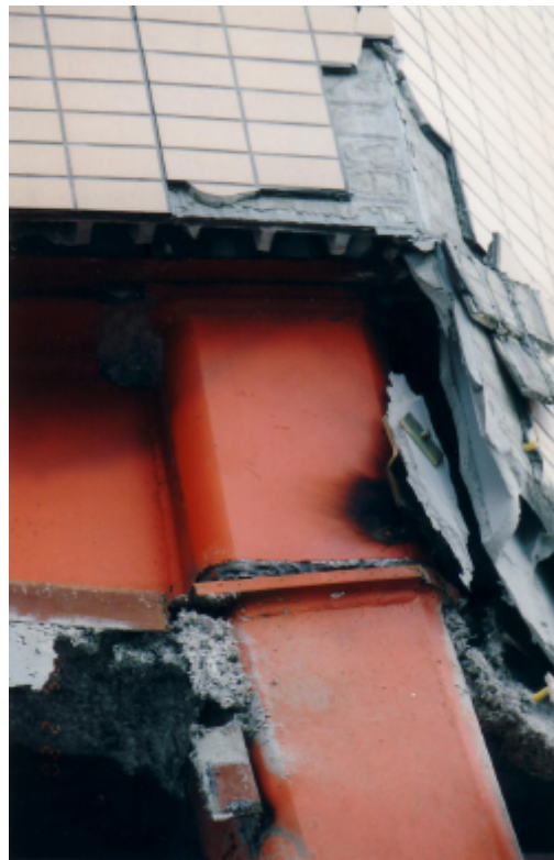
Photo 3.2.3-33 Rupture of a welded part between column and diaphragm
