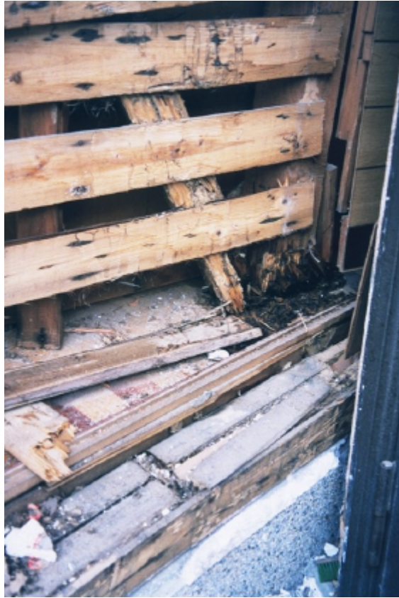
Photo 3.2.2-45 Ant damage (Rank C)
