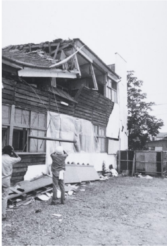
Photo 3.2.2-35 Differential settlement of a building (Rank C)
