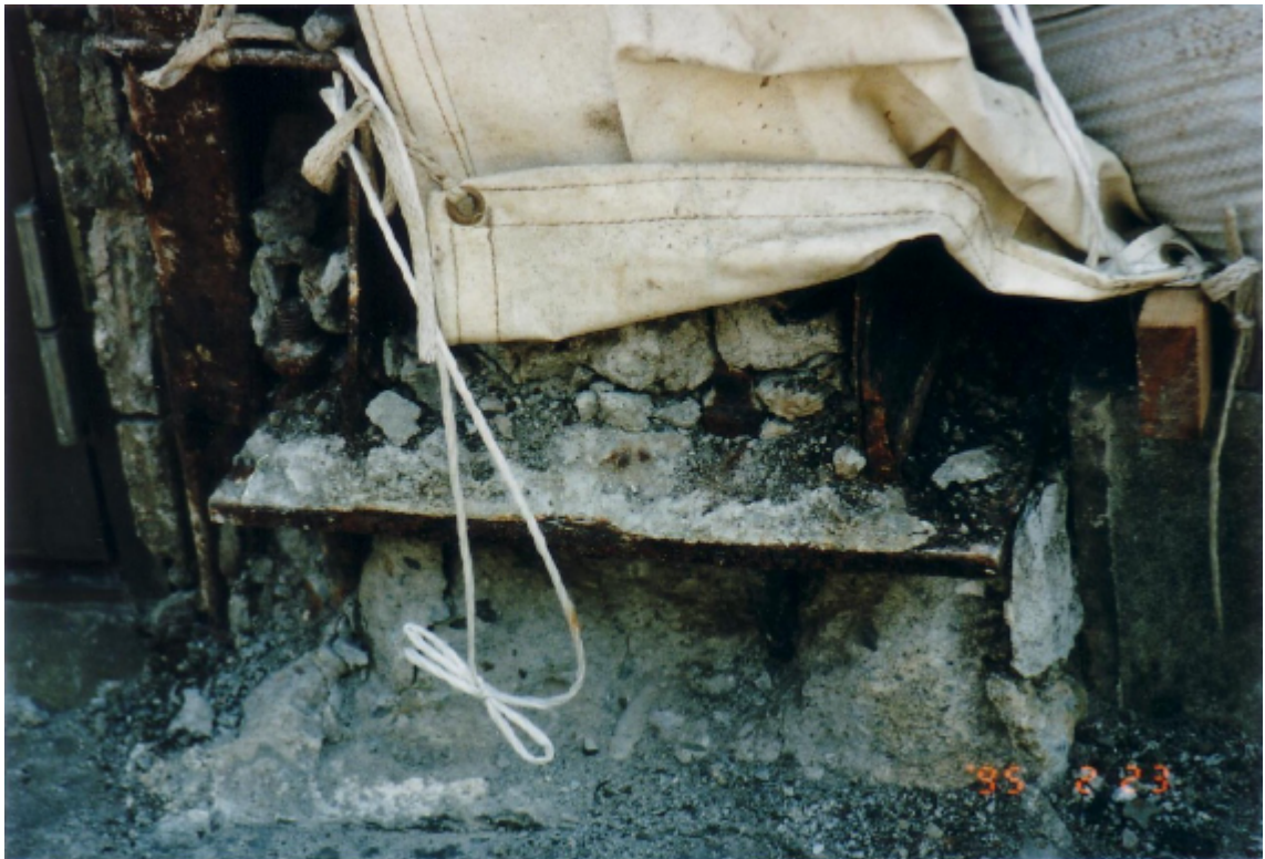
Photo 3.2.2-28 Concrete below a column base plate that has lost its axial load supporting capacity.
