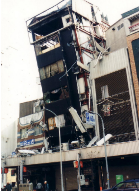
Photo 3.2.3-26 An inclined building
