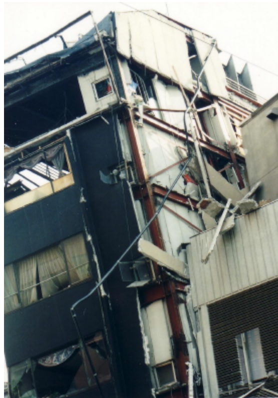
Photo 3.2.3-19 A building inclined to a large extent
