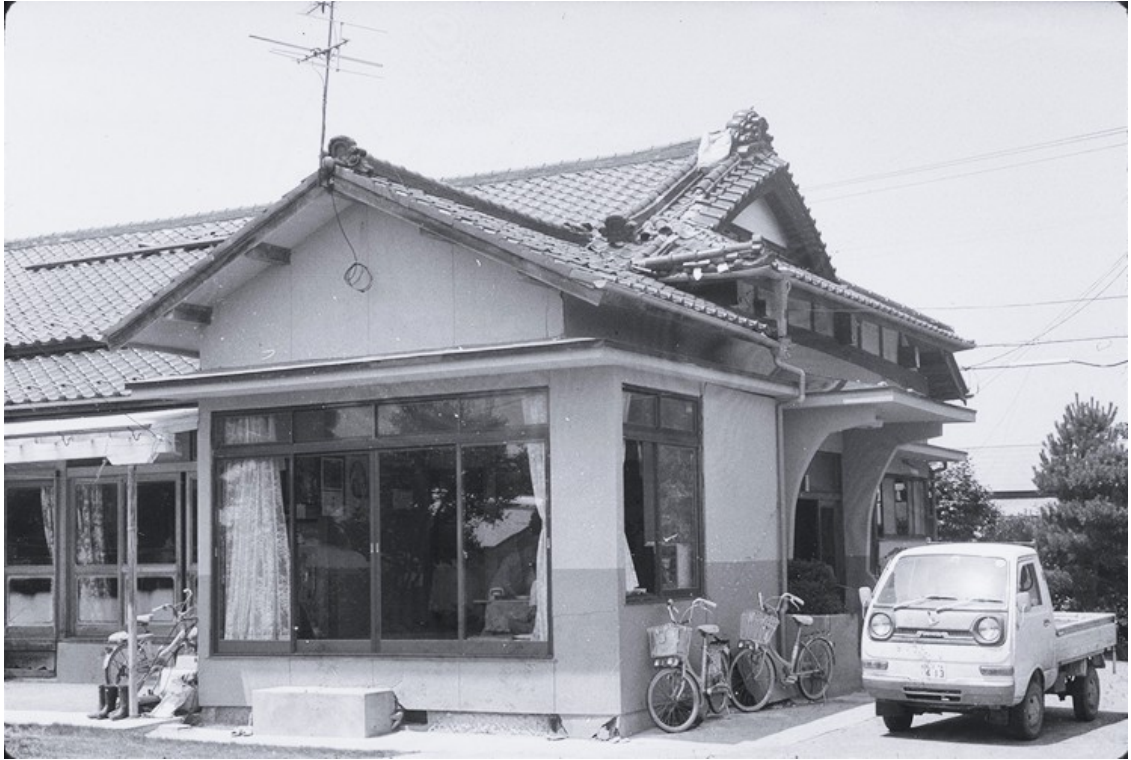
Photo 3.2.3-54 Slight damage This mono-color photo is produced by BRI members.
