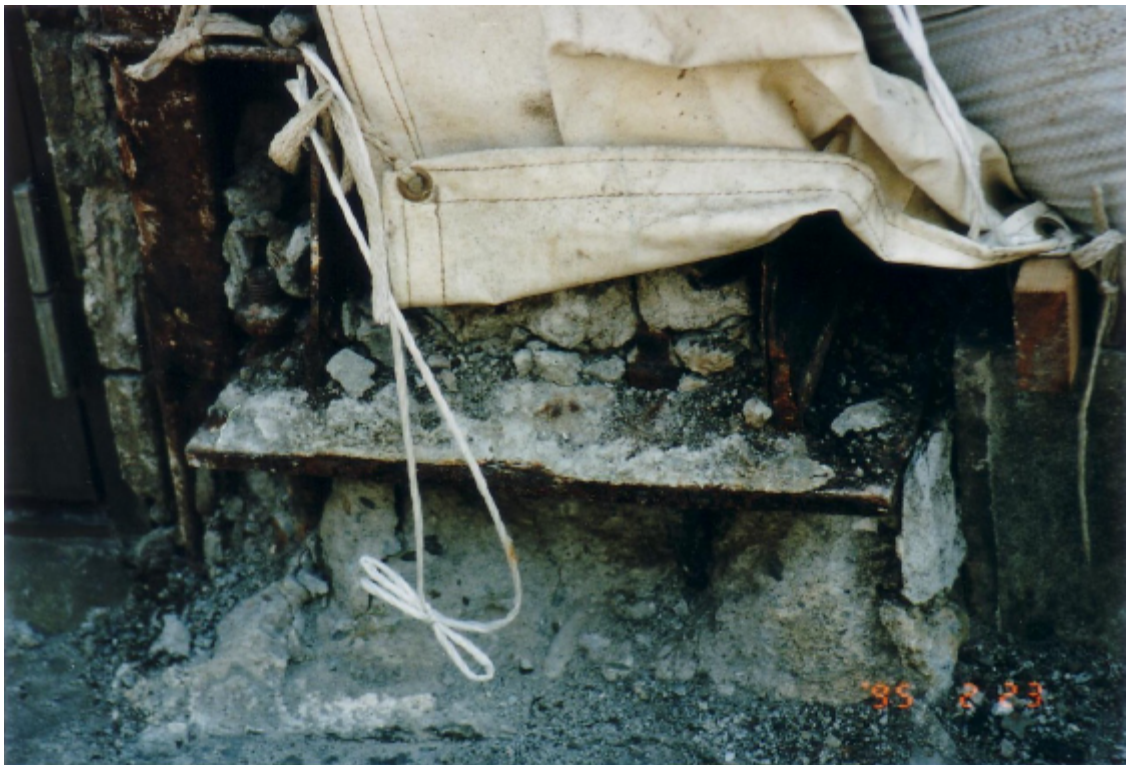
Photo 3.2.3-35 Concrete below a column base plate that has lost its axial load supporting capacity.
