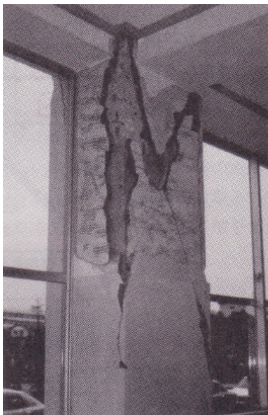
Photo 3.2.3-2 Covering concrete has come off to a large extent, but the column structure concrete has not come off much. The reinforcement is slightly exposed without deformation.
