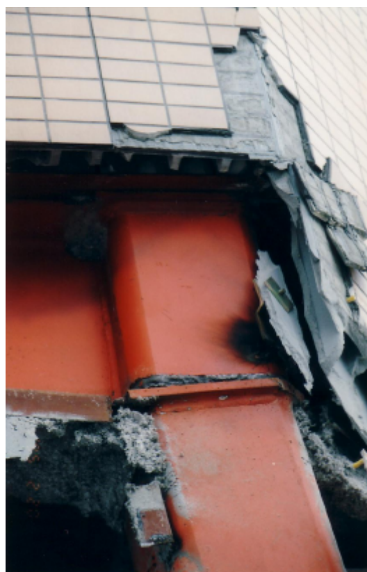
Photo 3.2.2-26 Rupture of a welded part between column and diaphragm
