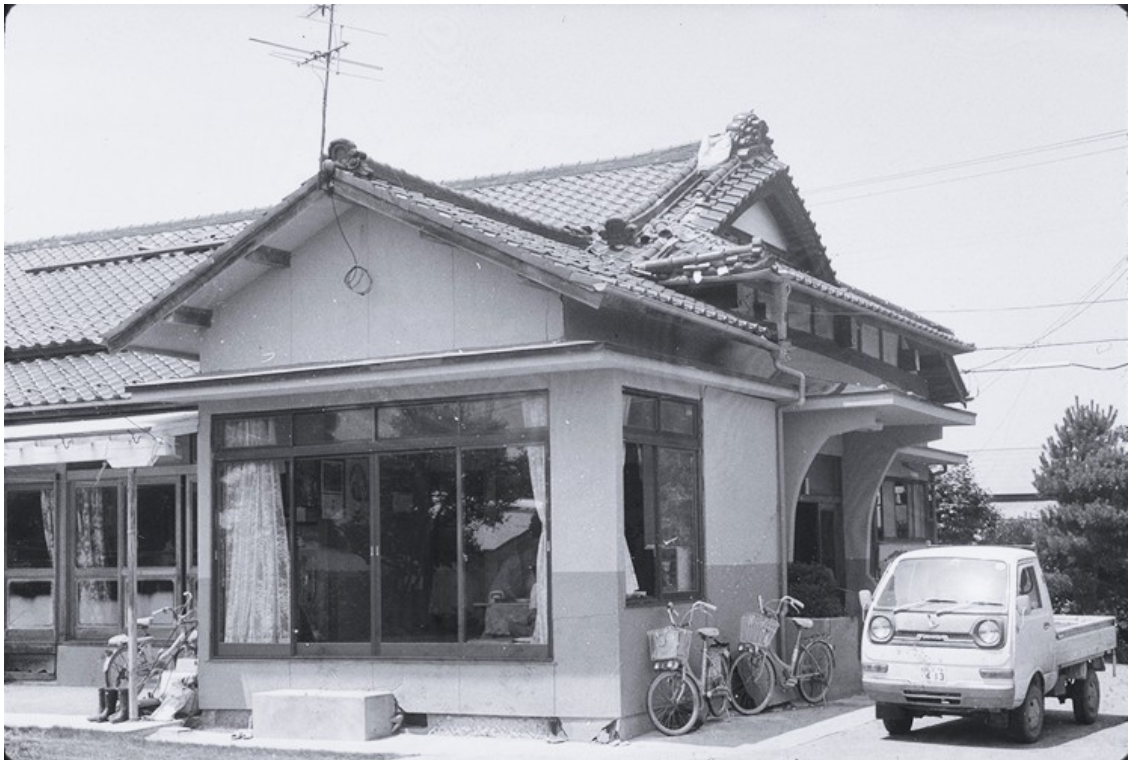
Photo 3.2.2-46 An object that can fall (roof tile) (Rank C)
