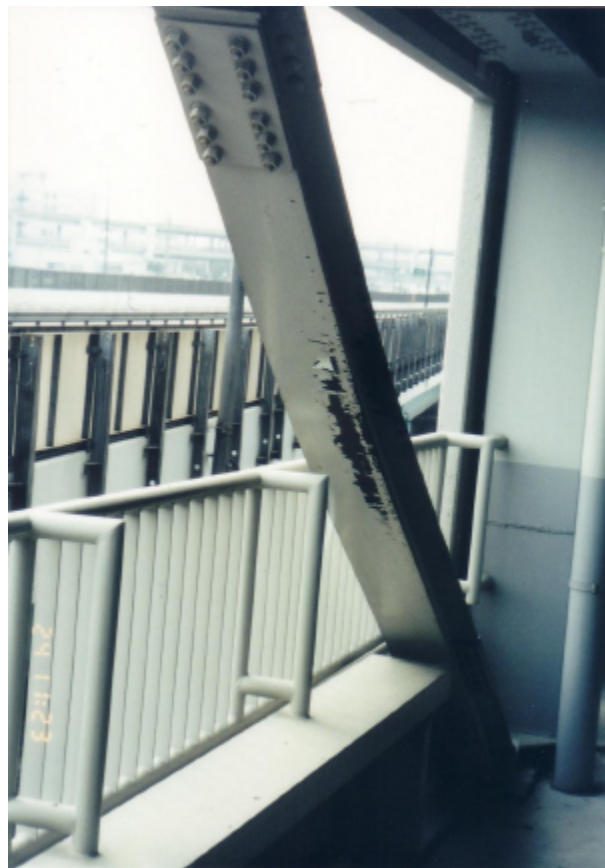
Photo 3.2.2-24 Buckling of wide-flange-shaped braces
