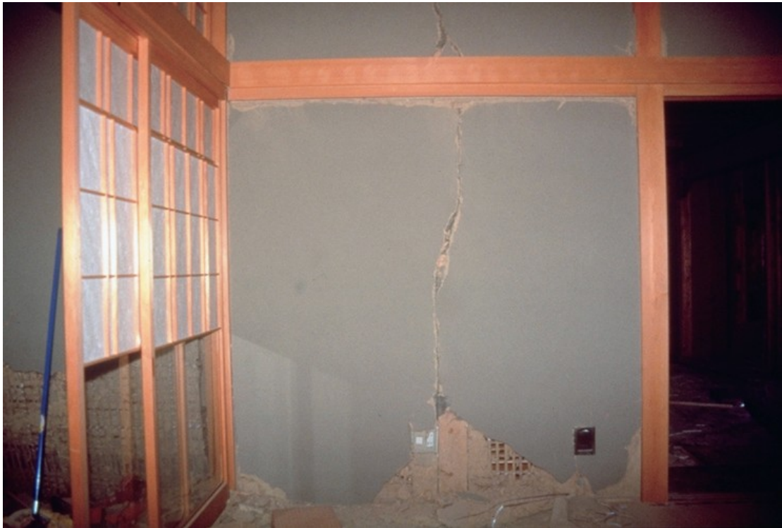
Photo 3.2.2-40 Damage on a wall (interior wall) (Rank B)
