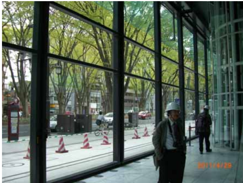
Temporary exterior glass for repair (3F)
