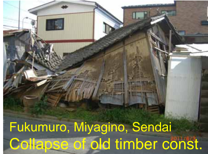
Failure of exterior walls
