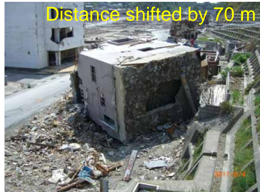
Pulled out friction pile
