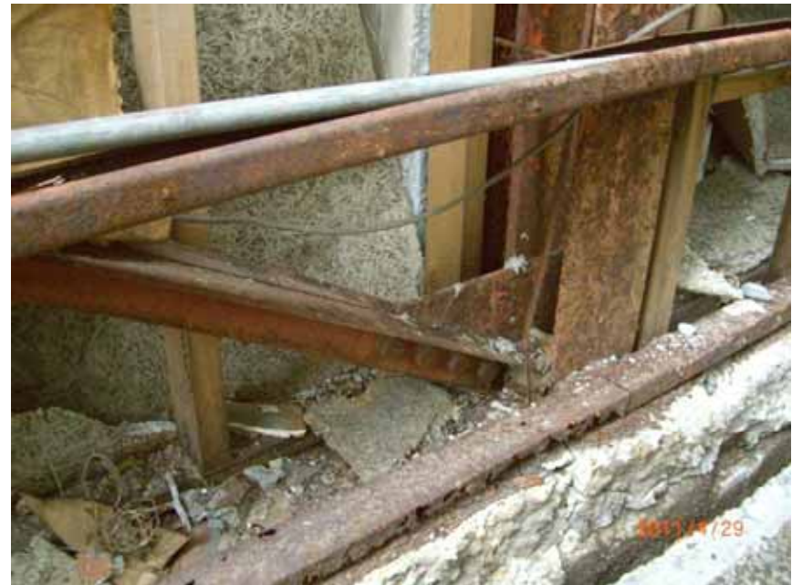
Net section fracture of gusset plate at brace end connection
