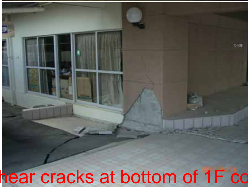
Shear failure of 1F nonstructural wall
