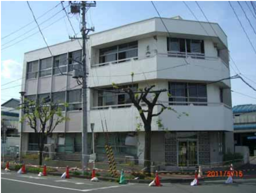
Higashimiyagino, Miyagino, Sendai Office, RC, 3F Shear failure of first story columns
