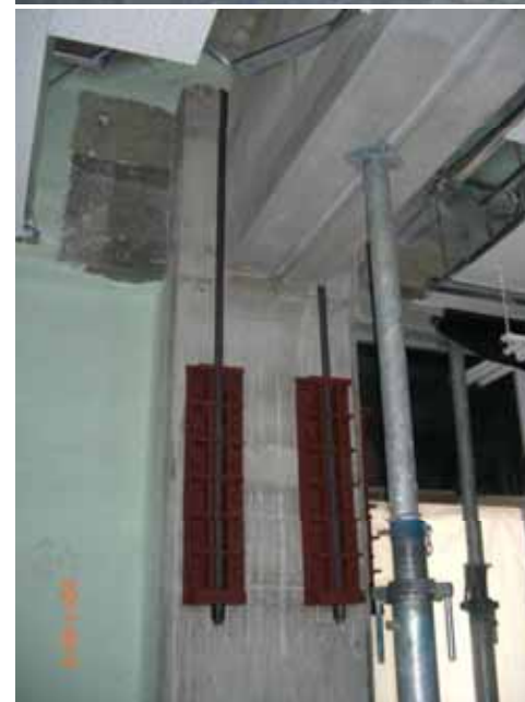
Tentative strengthening of crushed column (lower view)
