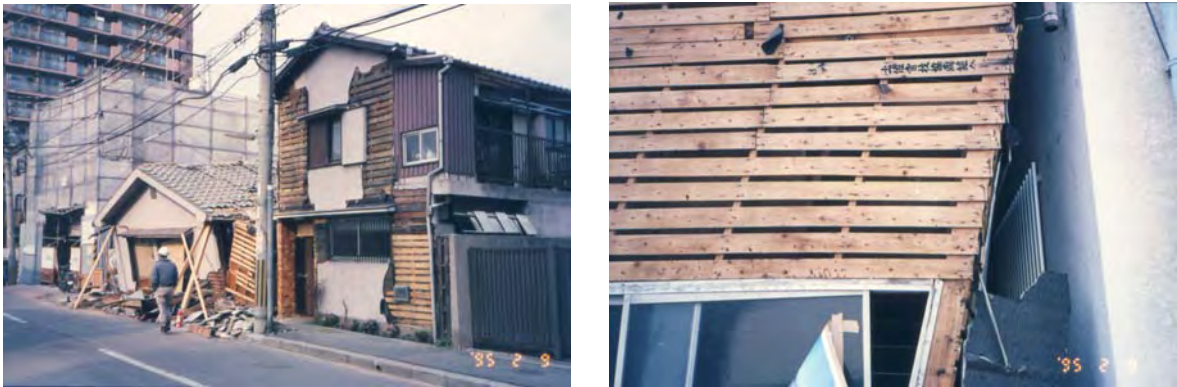
Figure 6.5: Damage to wooden houses (1995 Kobe Earthquake, Japan)
