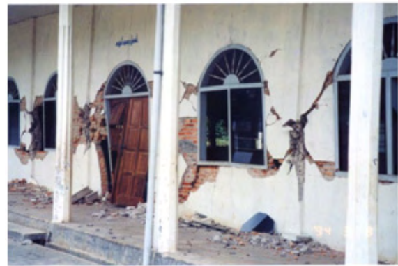
1994 Liwa earthquake, Indonesia
