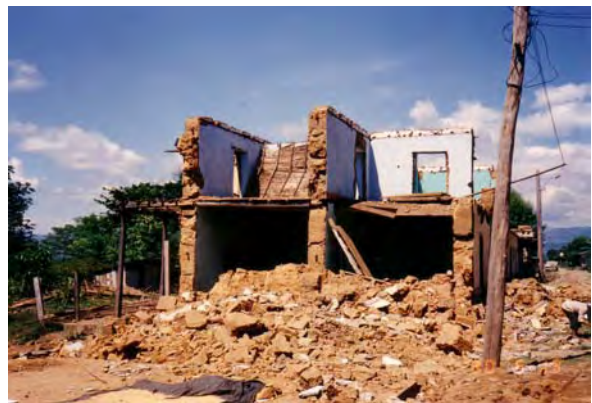
b) Damaged Tapial house
