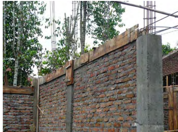
Two storey house under construction (Jawa, Indonesia)
