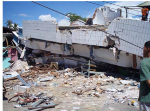
2009 West Sumatra Earthquake, Indonesia
