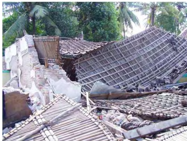
Figure 4.4: Damaged brick masonry (2006 Central Java Earthquake, Indonesia)
