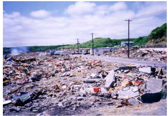
1993 Hokkaido-nansei-oki Earthquake, Japan (Tsunami run-up height reached 15 m average and 31 m max. and all houses were swept away.)
