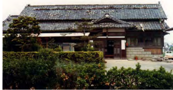
(Damaged wooden house in 1978 Miyagi-ken- oki Earthquake, Japan)
