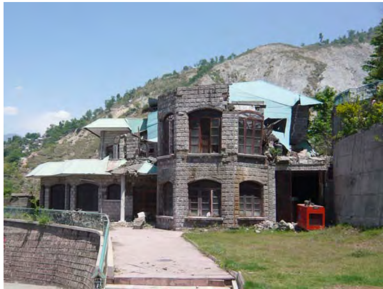
Figure 4.6: Damaged unreinforced masonry house (Muzafarabad, Pakistan) (2005 Northern Pakistan Earthquake)
