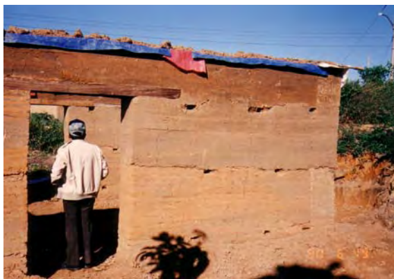
a) Tapial house under construction
