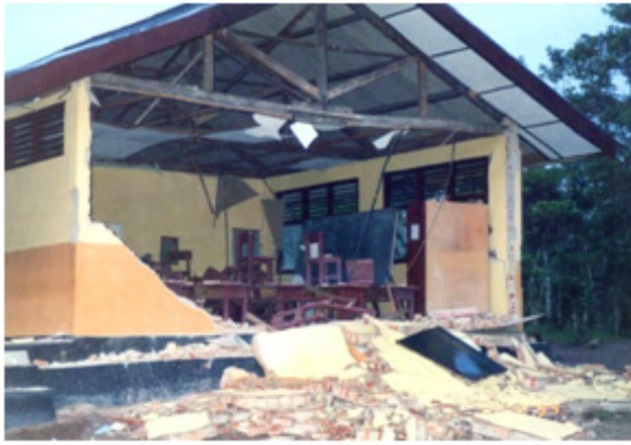
1994 Liwa Earthquake, Indonesia
