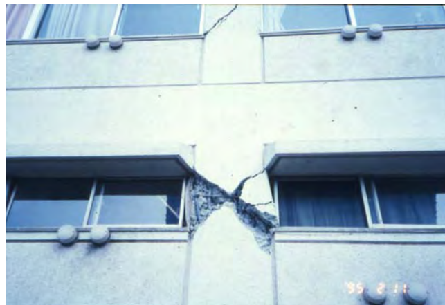
Figure 8.4: Diagonal shear cracks of a short column (1995 Kobe Earthquake, Japan)
