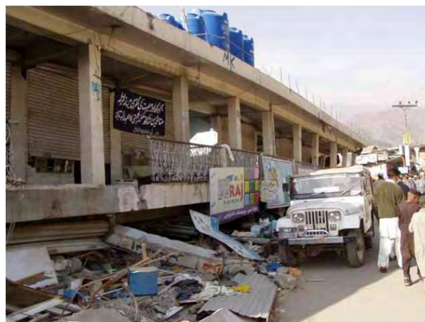
Figure 8.2: Collapsed RC building (2005 Northern Pakistan Earthquake)
