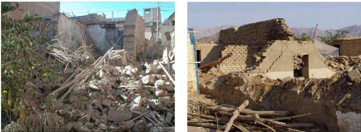
Figure 7.5: Damaged adobe (2007 Pisco Earthquake, Peru)
