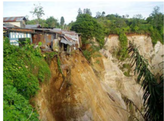
2007 West Sumatra Earthquake, Indonesia
