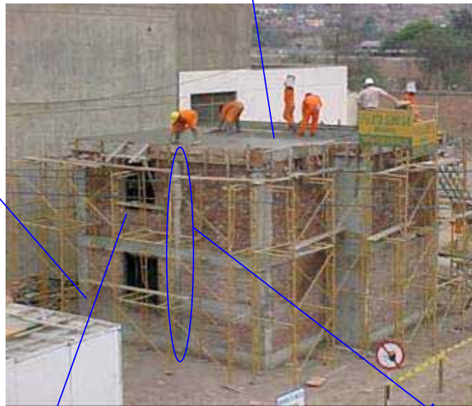
Detail of the Confined Column in its whole length.
