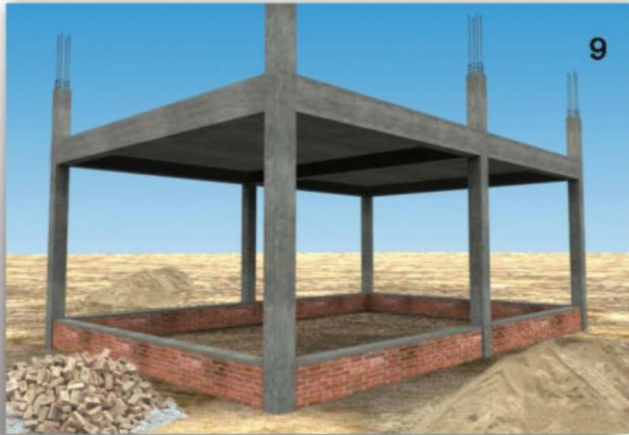
9. Fill concrete in the columns up to the lap level of 2 nd floor after fixing framework.
