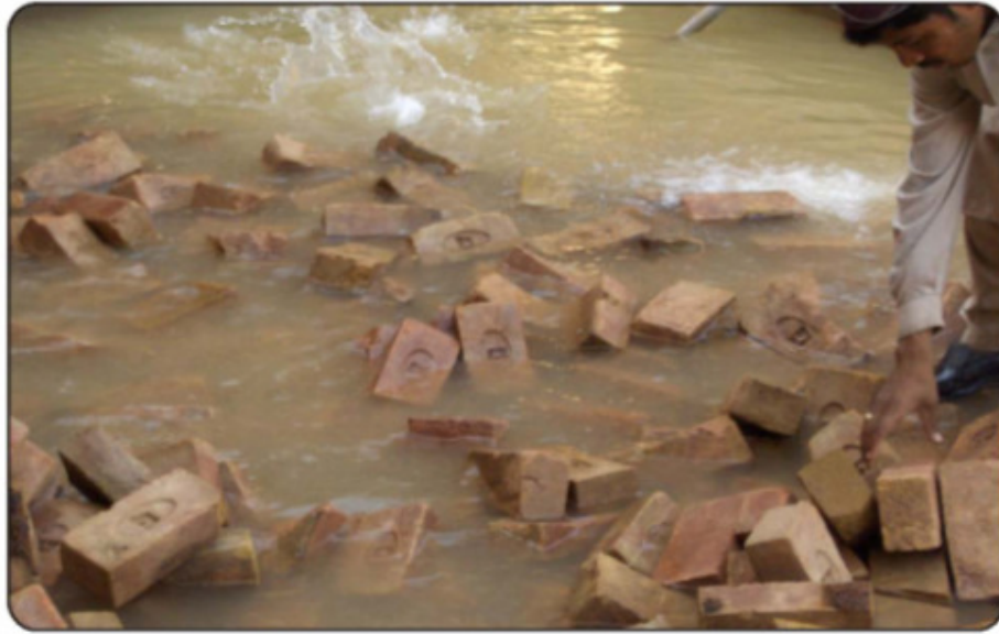
Fig.14 Soaking of bricks in water before use
