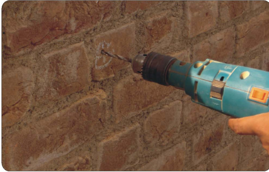
Fig.24 Drilling for fixing the mesh
