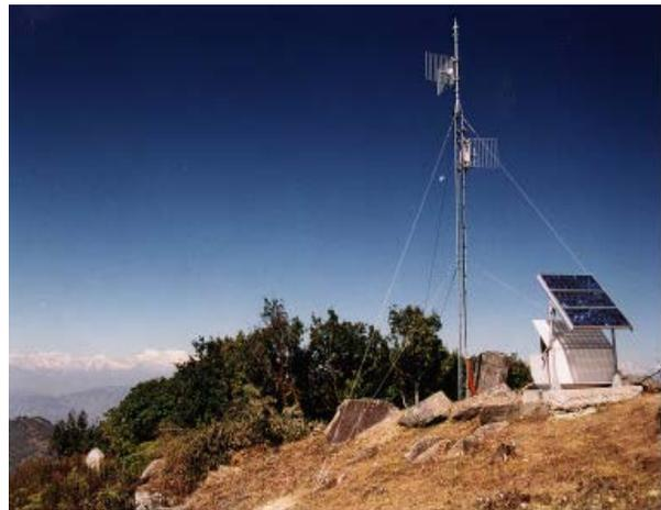
**Figure 3.** Typical Seismic Station
