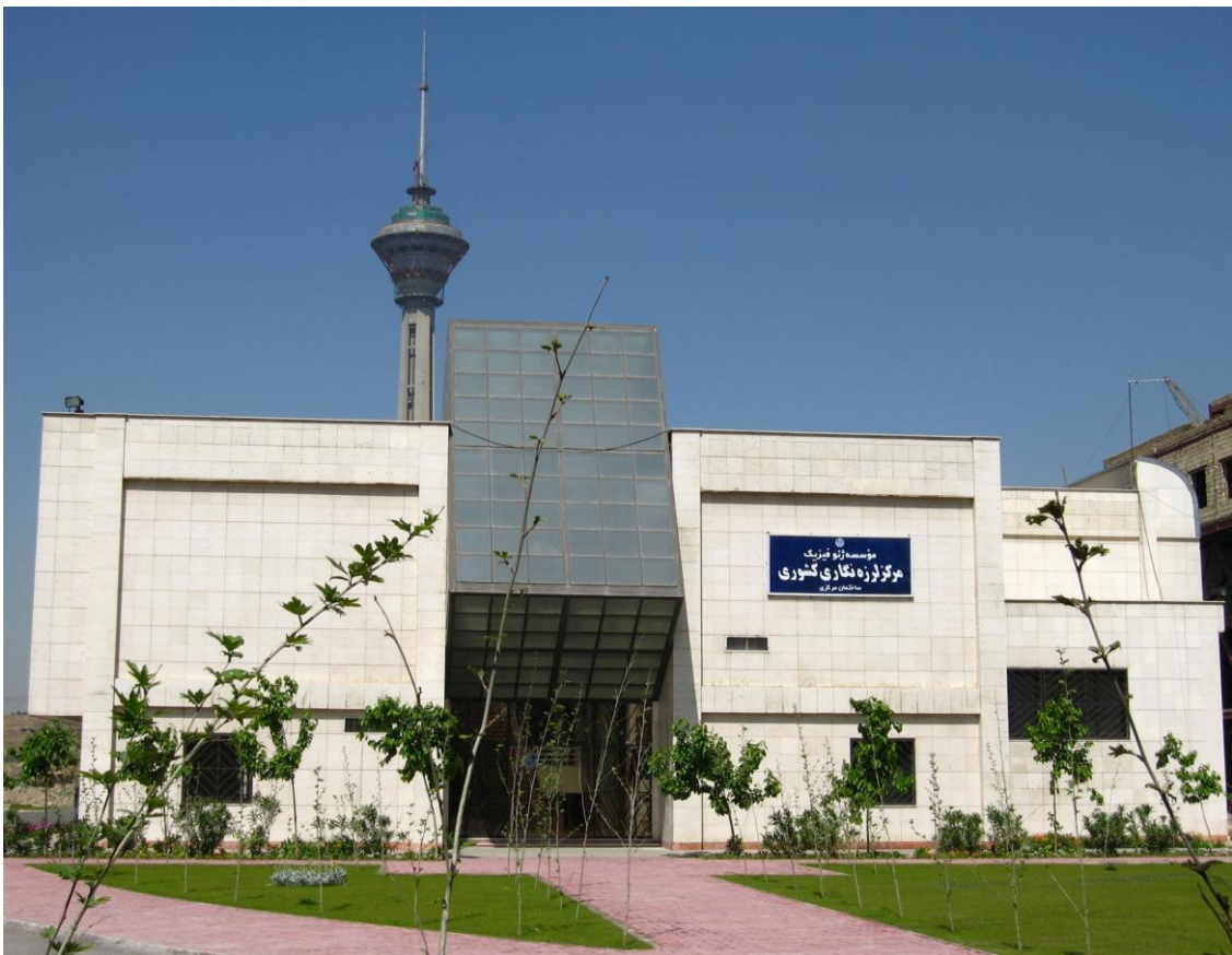
Figure 7. Building of IRSC.
