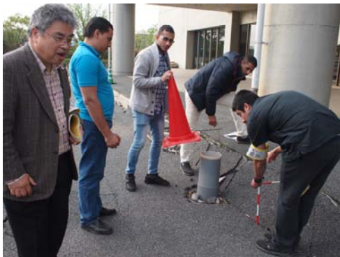
Liquefaction inspection in Mashiki in Kumamoto
