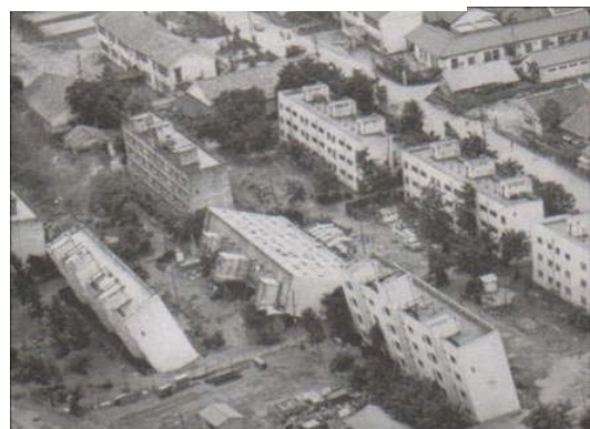
Photo 2. Liquefaction in 1964 Niigata Eq. (USGS)
