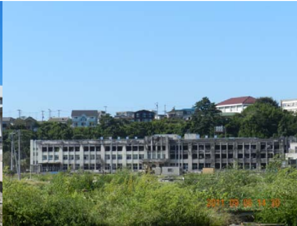
Photo 10. Kadowaki elementary school, completely destroyed, also due to fire.
