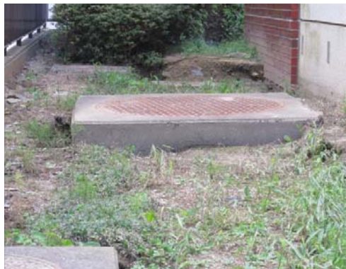
Photo 5. Outcropping RC water tank
