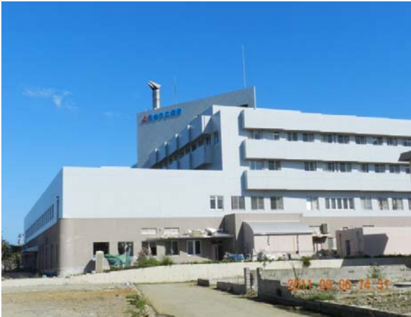
Photo 9. Hospital in Ishinomaki city severely damaged by earthquake and tsunami
