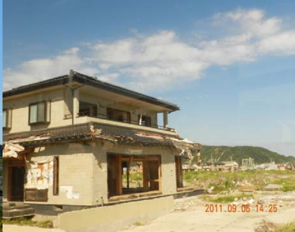
Photo 8. Severe damage caused by Tsunami to a wooden house in Ishinomaki city
