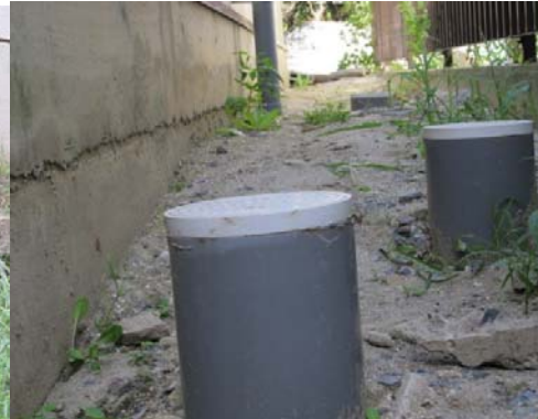
Photo 6. Outcropping steel facilities
