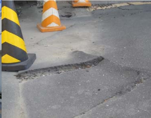
Photo 4. Out-of-flatness ground
