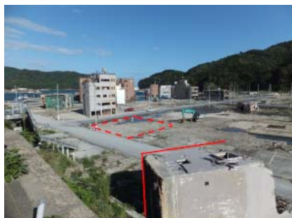
Figure 6. Drifted building with tsunami. It was drifted about 70 meters by the waves.
