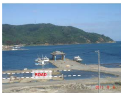
Figure 7. The old road near the port subsided about 80 cm.
