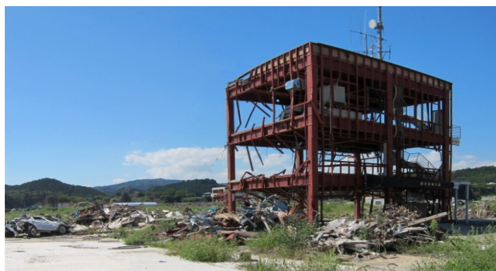
Figure 3. Disaster Management Center
