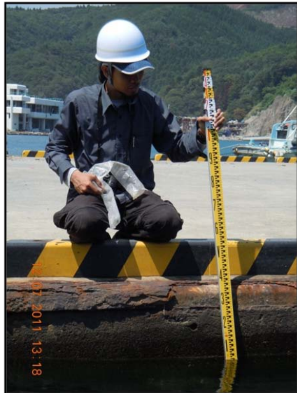
Figure 10: Because of subsidence, sea level is only about 35cm from the road. (Photo taken by Mazni Azis)
