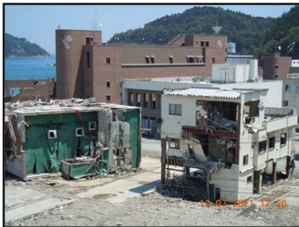
Figure 7: Heavily damaged buildings at Onagawa city (Photo taken by Mazni Azis)
