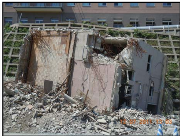
Figure 8: Building moved about 70m (Photo taken by Mazni Azis)
