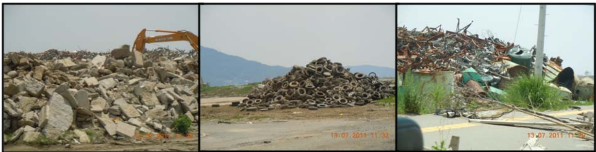
Figure 12: All debris is collected by type. (Photo taken by Mazni Azis)
