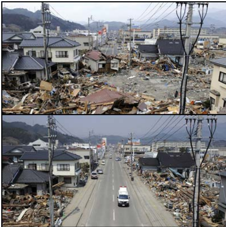
Figure 12: This pair of before-and-after photos shows the removal of tsunami destruction and debris covering the road in Ofunato city, Iwate prefecture on March 14, 2011, three-days after the tsunami disaster and after the road was cleaned of debris, on April 15, 2011. (Toshifumi Kitamura/AFP/Getty Images) http://www.theatlantic.com/infocus/2011/04/japan-earthquake-the-long-road-to-recovery/100047/#img24
