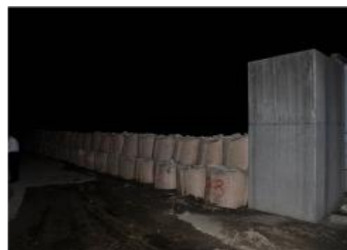
Figure 3.5. Temporary barrier to prevent overflow of sea water.
