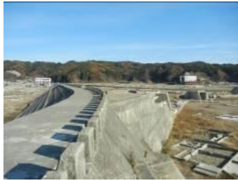
Figure 5.1. Embankment in Taro.
