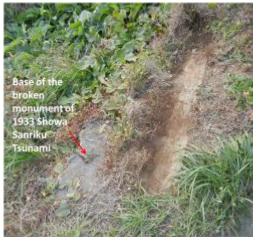
Figure 3.2. The broken monument of 1933 Showa Sanriku tsunami in Ofunato Bay.
