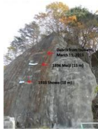
Figure 5.4. The previous tsunami water levels were mark on the rock.
