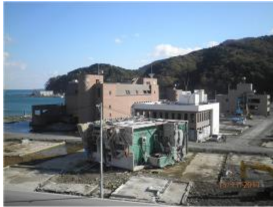
Figure 2.5. The collapsed RC building in Onagawa town. View from the evacuation point (15 m from the ground level).
