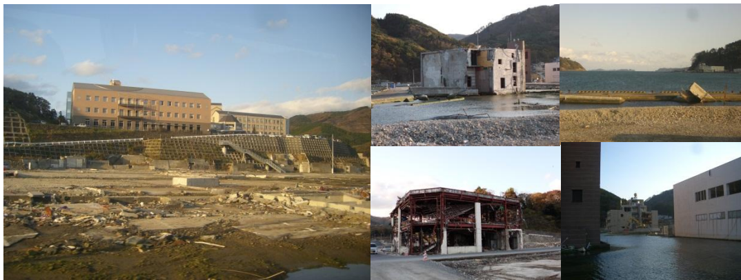
Figure 8. Heavily damaged buildings at Onagawa city
