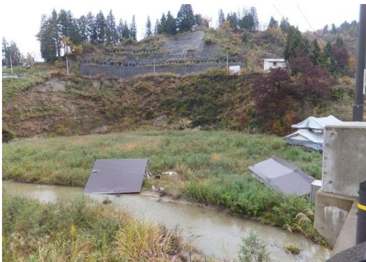
Figure 4. Landslide caused by the Chuetsu earthquake in Yamakoshi Village.
