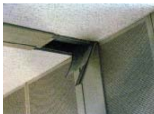
Fall of Cover at Expansion Joint
