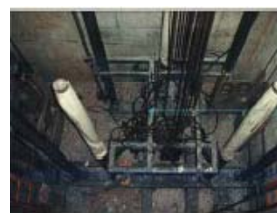
Tangled elevator cable
