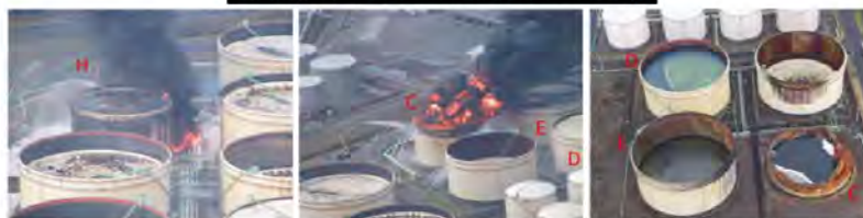
Damage due to the 2003 Tokachi-oki Eq.
