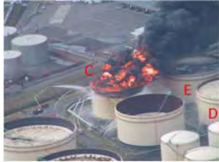
Open-Top Fire - Occurred 2 days later. - Lasted for 2 days.
