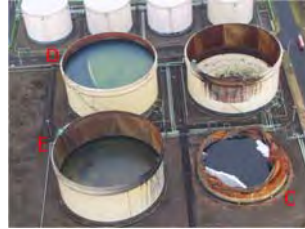
Sinking of the Floating Roof ➔ Oil Surface Exposed to the Atmosphere
