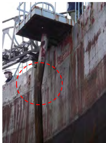
Deformation of the gauge pole (Wh-1.4 m)
