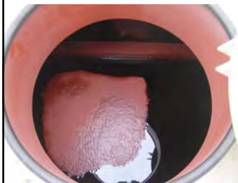
Infiltration of oil into pontoons (Wh-1.9 m)
