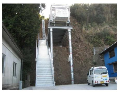
Tsunami Escape Station for a Millennium Tsunami at Yoshida Town, Shizuoka Prefecture. The construction was completed on 23<sup>rd</sup> September, 2013. Deck Height is 10.5 meters above mean sea level. This place of refuge can accommodate 1,000 people.
