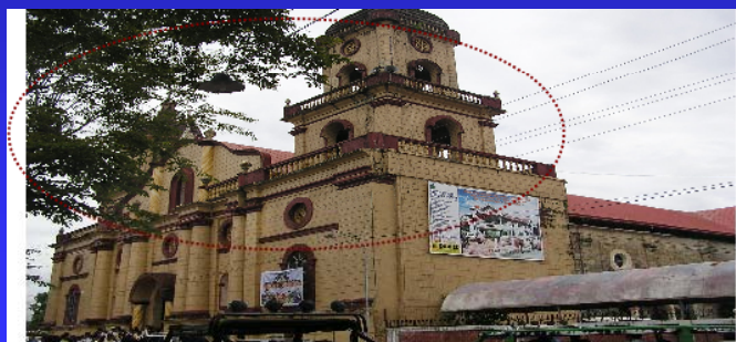
Photo of damage Courtesy of Lambunao Fiesta Program
