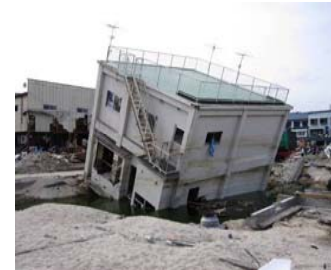
Mat foundation (直接基礎)
