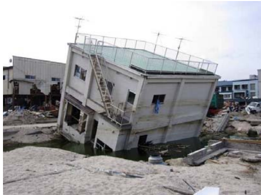
A building with mat foundation tilted due to scouring (洗掘により直接基礎の建築物が傾斜した例)
