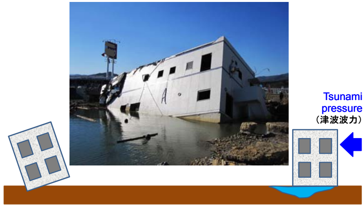
Pile foundation is effective to prevent sliding (滑動防止には杭基礎が有効)
