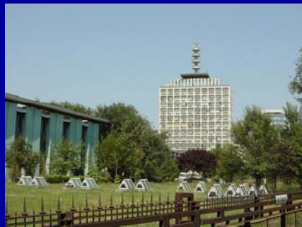
National Romanian Television. RC frame structure built before 1977 earthquake (14 storeys)
