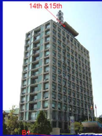
National Romanian Television. RC frame structure built before 1977 earthquake (14 storeys)
