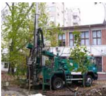
Figure 3. Drilling equipment on truck
