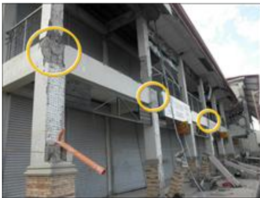
Figure 18 An example of improper rebar works in Market Building in Loon (by the earthquake): (Left) Failures at panels, (Right) Detail of damaged part
