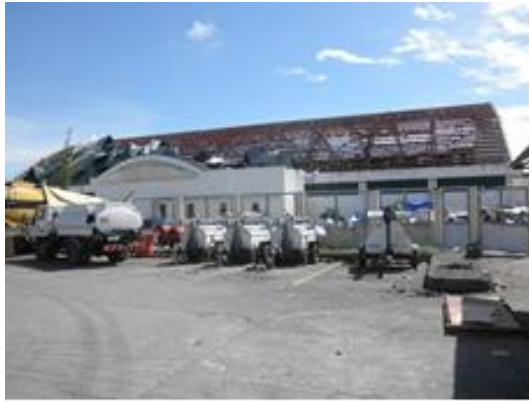
Figure 7 Typical damage by strong winds by the typhoon: (Left) Heavy damage in roofing: Customers' center of private company in Palo, Leyte, (Right) Damage to both roofing and roof trusses. Sagkahan National High school, Tacloban, Leyte
