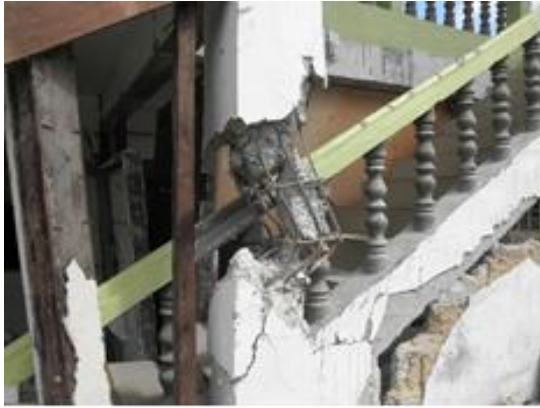
Figure 20 Examples of improper rebar works (by the earthquake): (left) Barangay Office in Antequera, (Right) A building under construction, Basey National High School
