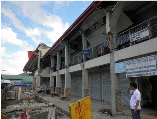
Figure 17 Examples of improper rebar works in Market Building in Loon (by the earthquake): (Left) Heavy damage at the bottom of most of columns, (Right) Detail of the damage.
