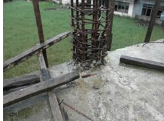
Figure 20 Examples of improper rebar works (by the earthquake): (left) Barangay Office in Antequera, (Right) A building under construction, Basey National High School
