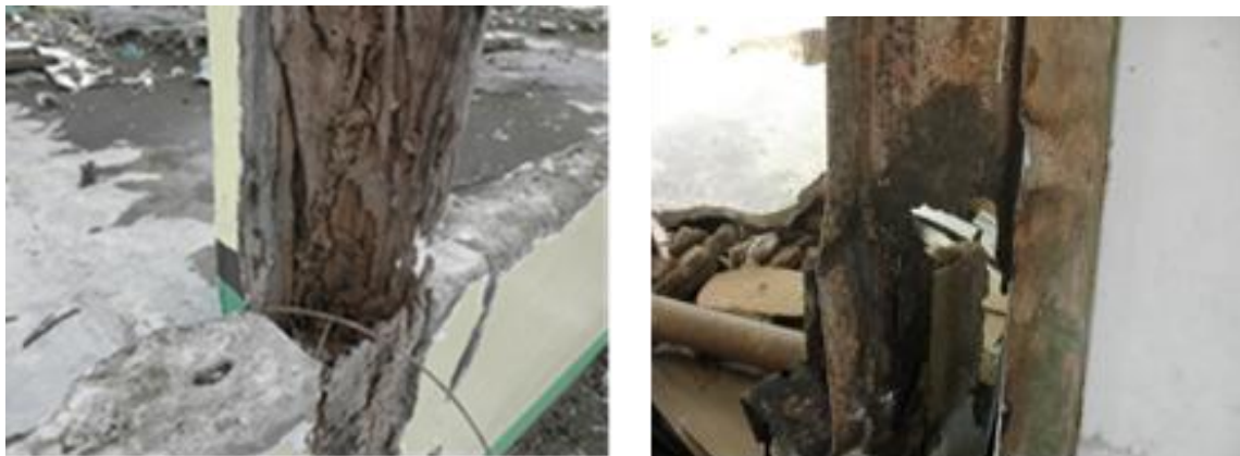
Figure 24 Examples of failures by lack of maintenance: (Left) St. Joaquin Central Elementary School, Palo, Leyte (by the typhoon), (Right) Cogon Norte Elementary School, Loon, Bohol (by the earthquake)
