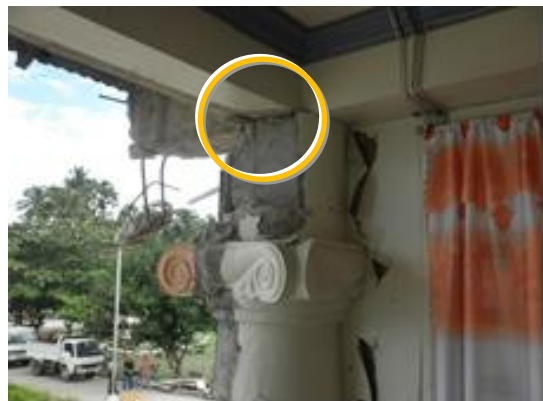
Figure 19 Examples of improper concrete placing (by the earthquake): (left) Market Building in Loon, (Right) Sagbayan Municipal Office
