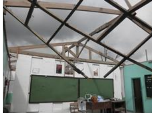
Figure 7 Typical damage by strong winds by the typhoon: (Left) Heavy damage in roofing: Customers' center of private company in Palo, Leyte, (Right) Damage to both roofing and roof trusses. Sagkahan National High school, Tacloban, Leyte
