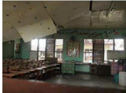
Figure 25 Examples of damage by inundation (by the typhoon): (Left) Basey National High School, Samar, (Right) Sagkahan National High School in Tacloban, Leyte
