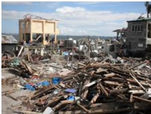
Figure 8. Typical damage by storm surge caused by the typhoon in coastal area of Tacloban city, Leyte
