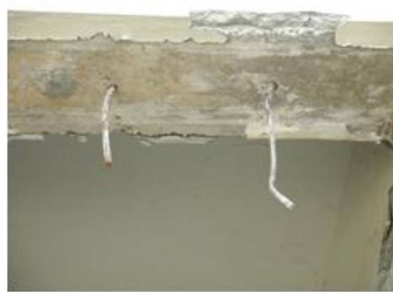
Figure 21 Examples of improper anchorage of CHB walls to RC members in Market Building of Loon (by earthquake): (Left) a case of horizontal rebar, (Right) a case of vertical rebar
