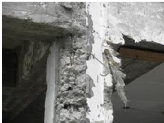
Figure 19 Examples of improper concrete placing (by the earthquake): (left) Market Building in Loon, (Right) Sagbayan Municipal Office
