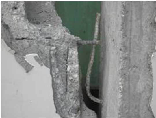
Figure 21 Examples of improper anchorage of CHB walls to RC members in Market Building of Loon (by earthquake): (Left) a case of horizontal rebar, (Right) a case of vertical rebar
