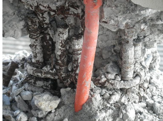
Figure 17 Examples of improper rebar works in Market Building in Loon (by the earthquake): (Left) Heavy damage at the bottom of most of columns, (Right) Detail of the damage.
