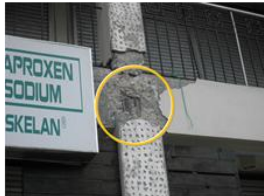
Figure 18 An example of improper rebar works in Market Building in Loon (by the earthquake): (Left) Failures at panels, (Right) Detail of damaged part
