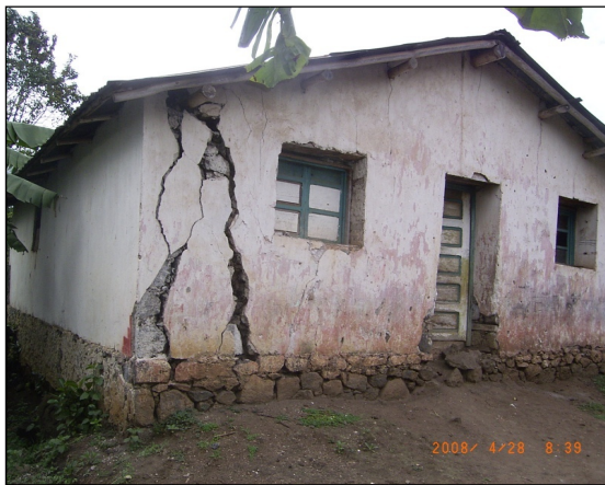
Fig.11a Wide vertical fissures observed on the wall at Kankule (D.R.C.), Apr. 28, 2008, (©Wafula)
