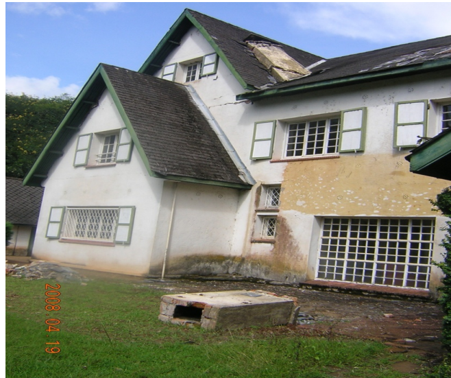
Fig. 10 The collapse of the chimney of house at Birava (the closest town to the epicentre area) Apr. 19, 2008 (©Wafula)
