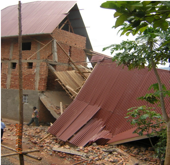
Fig. 9a Collapsed house with three floors, Bukavu city (Feb. 7, 2008) (©Wafula)
