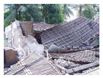
Figure 4.4: Damaged brick masonry (2006 Central Java Earthquake, Indonesia)
