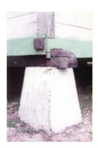
Figure 3.4: "Traditional" isolation (Sukabumi, Indonesia) (This may not prevent the house falling off its piers in a moderate and large earthquake.)
