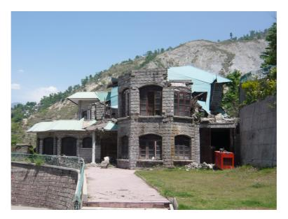
Figure 4.6: Damaged unreinforced masonry house (Muzafarabad, Pakistan) (2005 Northern Pakistan Earthquake)
