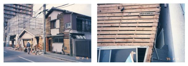
Figure 6.5: Damage to wooden houses (1995 Kobe Earthquake, Japan)
