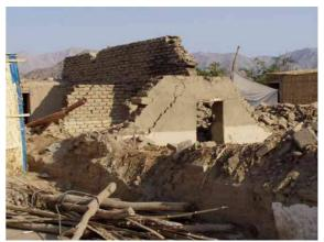
Figure 7.5: Damaged adobe (2007 Pisco Earthquake, Peru)
