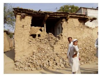
Figure 5.4: Damage to stone masonry (2005 Northern Pakistan Earthquake)
