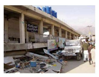
Figure 8.2: Collapsed RC building (2005 Northern Pakistan Earthquake)
