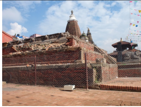
Photo 2: Microtremor observation at the Patan Durbar Square
