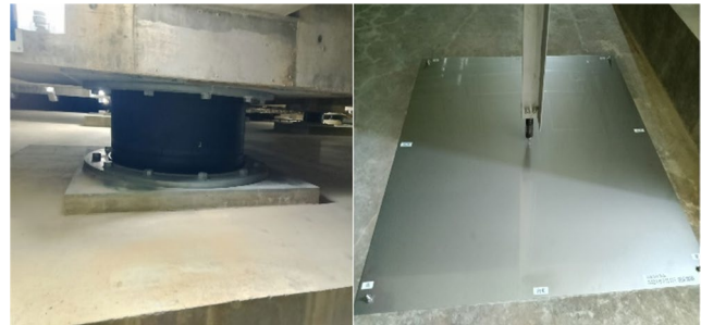
Picture 1: Seismic isolation device and sketch board to measure seismic response of isolation system at Keiju Medical Center
