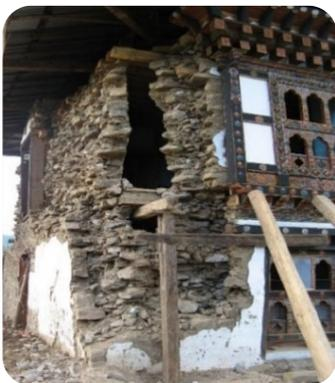
Figure 1. Damage pattern of stone masonry houses due to earthquake in Bhutan. The failure shows in-plane, out-of-plane and missing the key components like cornerstones and bonding stones.
