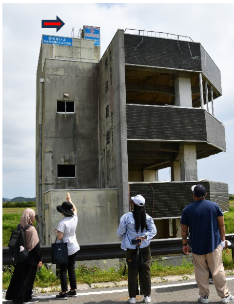
Photo of Yonezawa Shokai building showing 2011 tsunami surge height at the site, which remains as an educational landmark .
