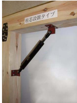
Joint oil damper for wooden house
