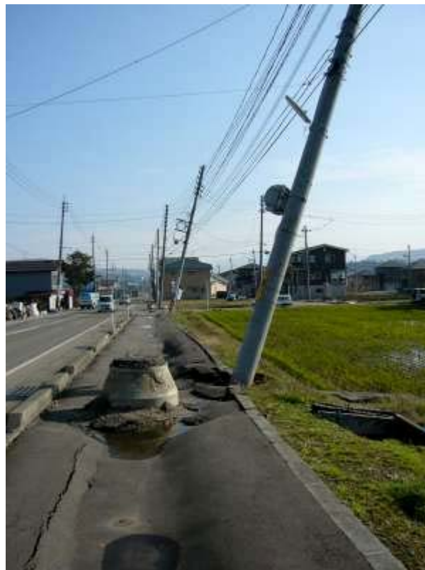
Ojiya, liquefaction of soils.
