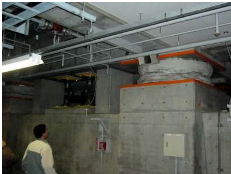
Rubber bearing and lead damper.
