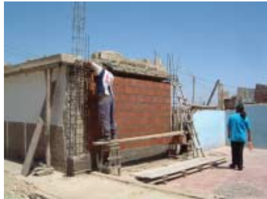
Picture 2-3-5-4. Repair work nearby.
