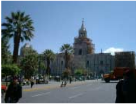
Picture 2-1-7-1. Full view of the Cathedral. The left tower has collapsed. The right-hand tower, which just escaped collapse, under repair at the time, was reinforced with scaffolding.
