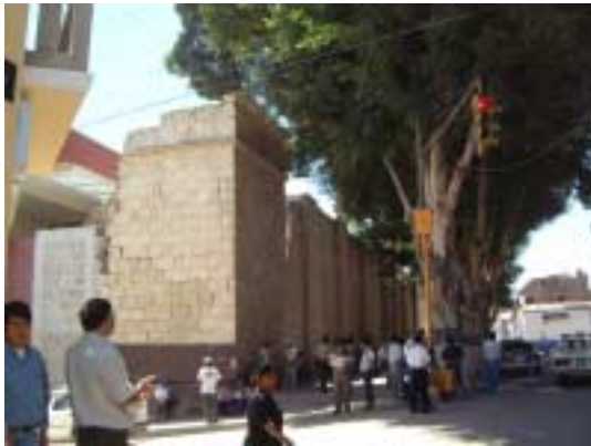
Picture 2-2-6-1. Full view of the wall.
