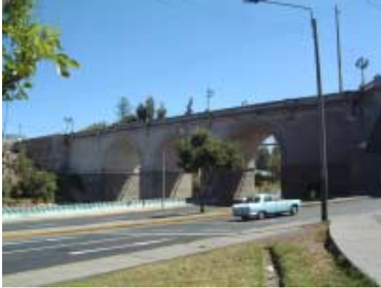
Picture 2-1-6-1. A bridge near Centro. Masonry arched bridge.
