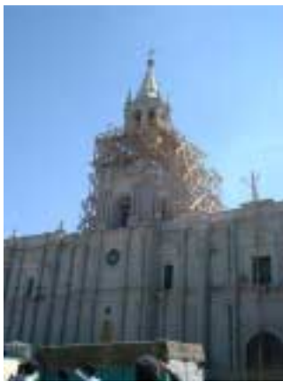
Picture 2-1-7-2. Tower under repair.
