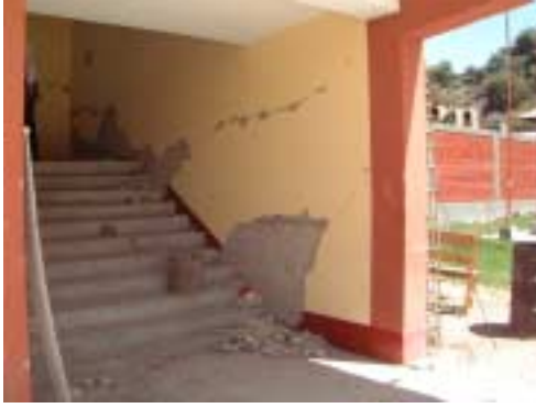
Picture 2-2-4-4. Brick wall of the staircase.
