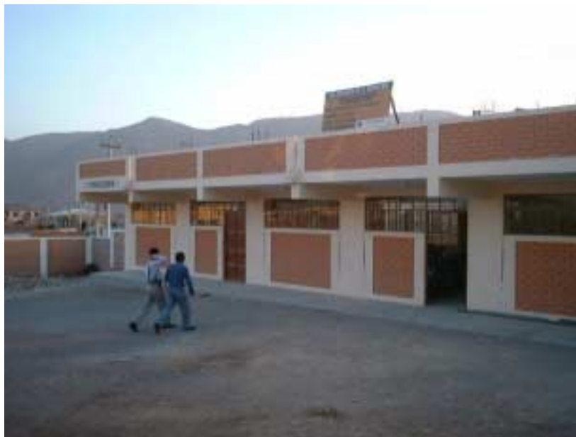
Picture 2-1-5-1. Full view of the building constructed in 1995. It was intact.
