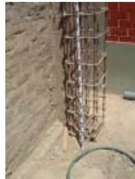
Picture 2-2-4-7. Bar arrangement of the extended part.
