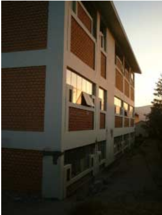
Picture 2-1-5-2. Full view of the schoolhouse constructed in 1993.
