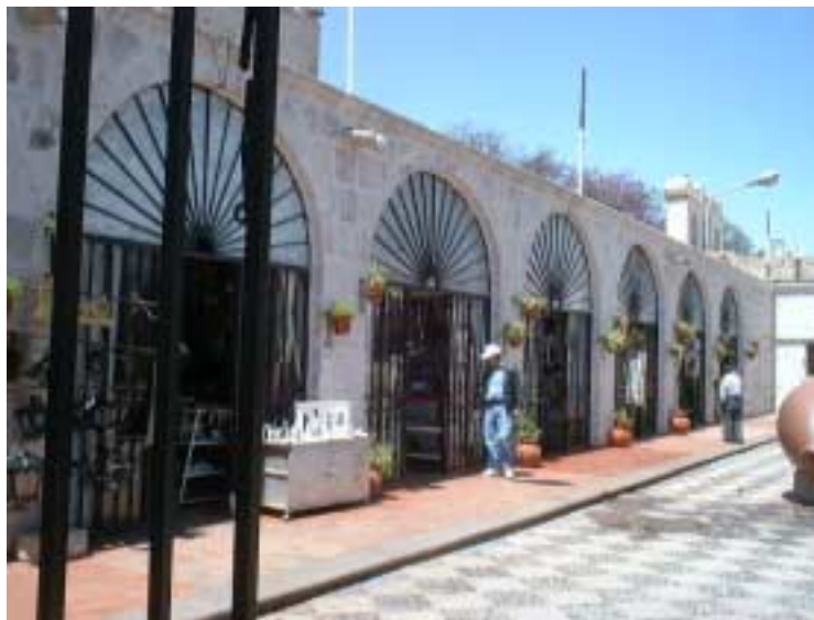
Picture2-1-9-2. Sillar blocks were used as structural elements.
