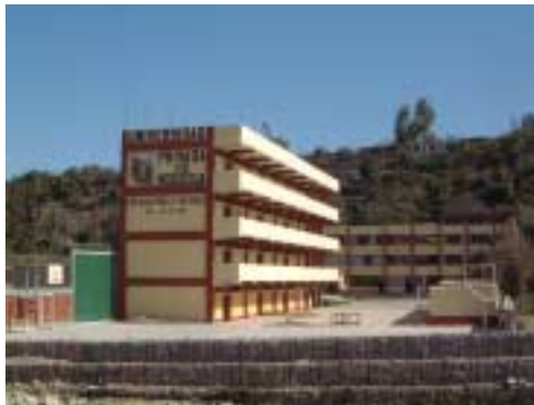
Picture 2-2-4-1. Appearance of the building.
