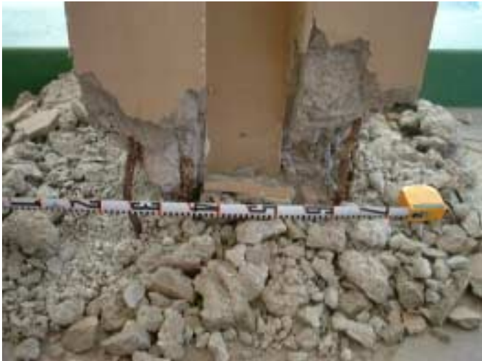
Picture 2-2-9-4. Column base. Reinforcements are jointed at the terminal (right terminal).
