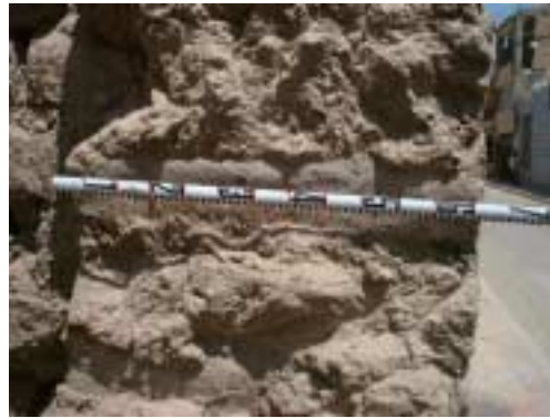
Picture 2-2-5-4. Unit length of an adobe block.
