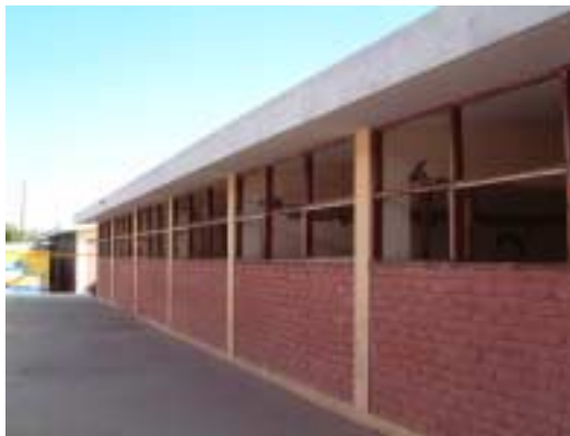
Picture 2.1.2-1. Appearance of schoolhouse. One-storied, brick spandrel wall.
