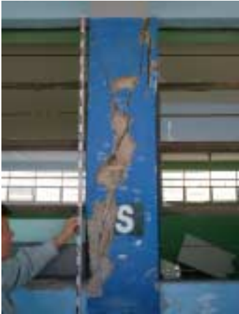
Picture 2-3-4-3. The length of the compressed column was about 145 cm.
