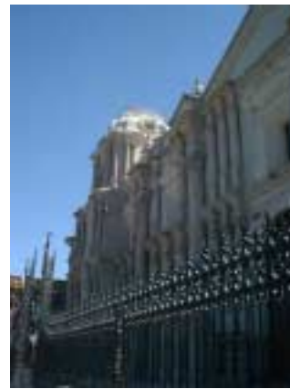
Picture 2-1-7-3. Partially collapsed tower.
