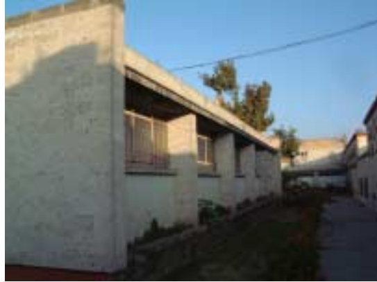
Picture 2-1-4-4. New masonry building.
