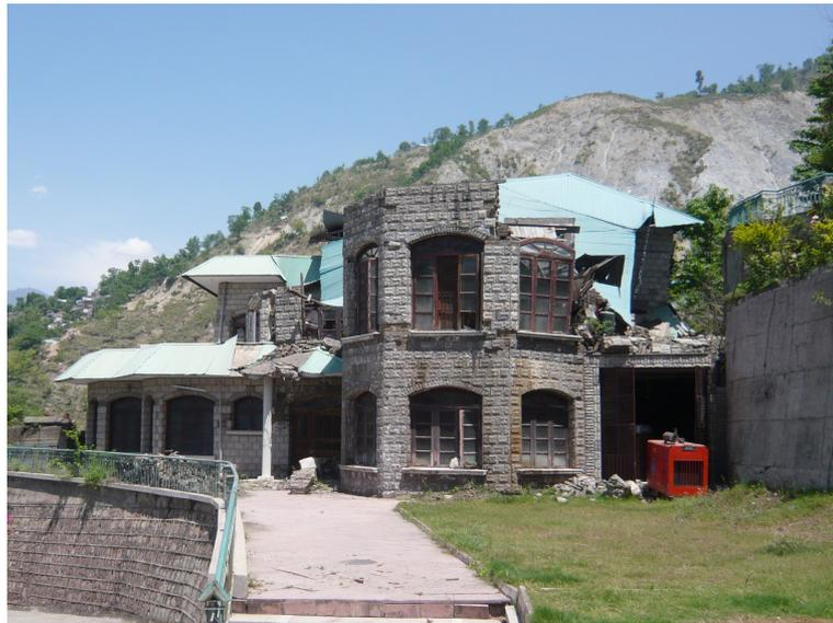
Figure 4.6: Damaged unreinforced masonry house (Muzafarabad, Pakistan)
