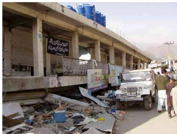
Figure 8.2: Collapsed RC building
