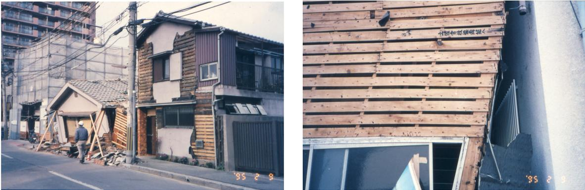
Figure 6.5: Damage to wooden houses (1995 Kobe Earthquake, Japan)
