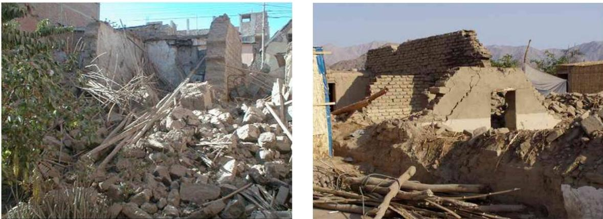
Figure 7.5: Damaged adobe (2007 Pisco Earthquake, Peru)
