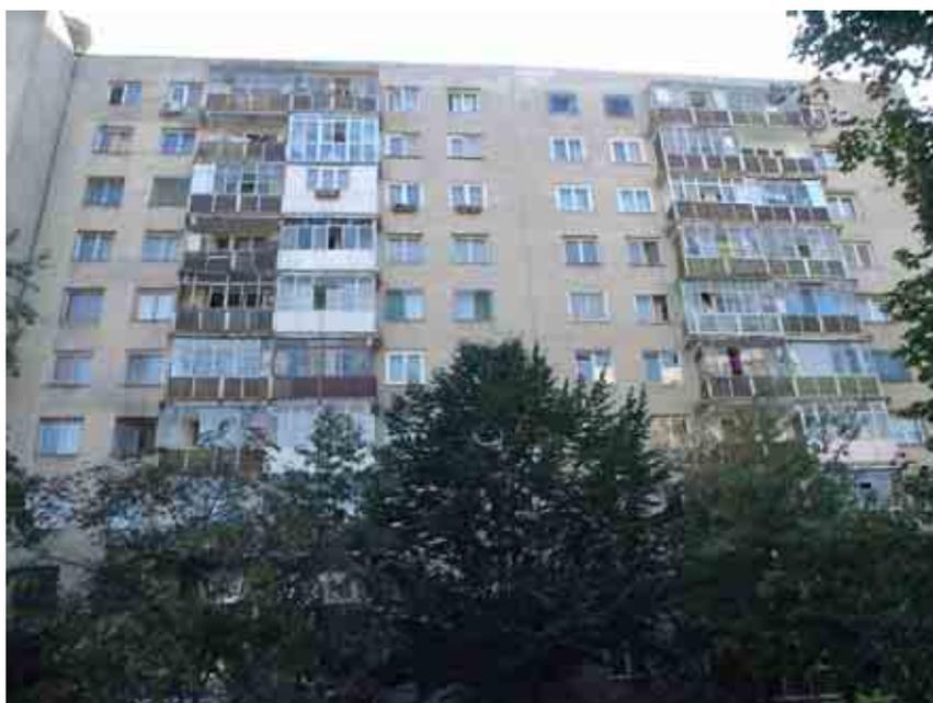
Figure B.2. Typical RC shear wall apartment building
