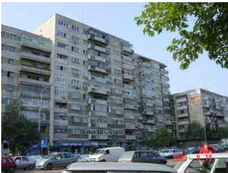
Figure B.1. Typical RC frame apartment building, built in 80's
