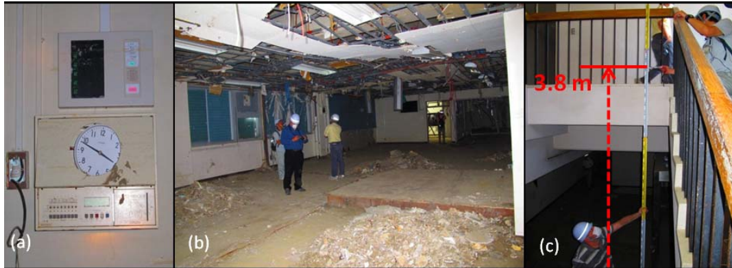
(a) Clock stopped due to tsunami; (b) all the ceilings collapsed; (c) tsunami water height reached the second floor with height of 3.8 m.
