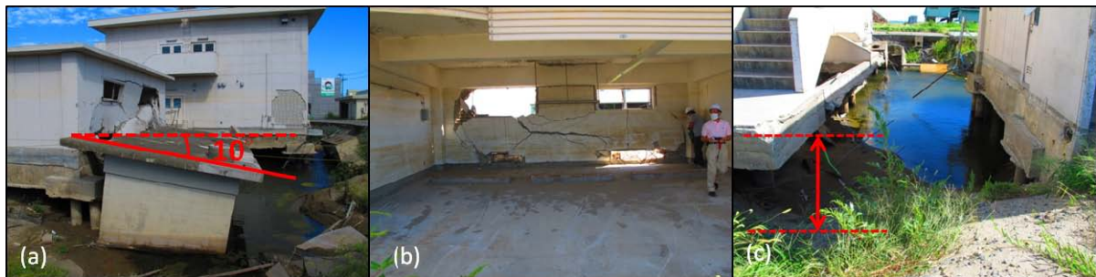
(a)The affiliated building was seriously damaged by tsunami; (b) Front view of the affiliated building; (c) Scouring caused by earthquake.
