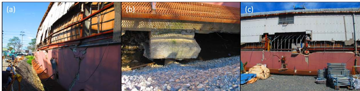
(a) Side view of a warehouse; (b) the basement cracked and rotated; (c) Front view of the warehouse.
