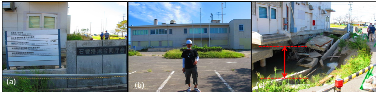
(a)The gate of Ishinomaki harbor combination government building; (b) Front view of the building; (c) Side view, collapsed fence, and the building subsided due to scouring.
