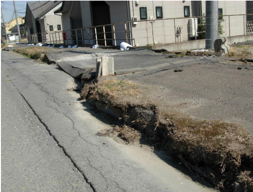
Photo 9. Distortion of the ground surface. The sidewalk went up and the road went down, crack at the road, this is clear evidence of the occurrence of liquefaction phenomenon.
