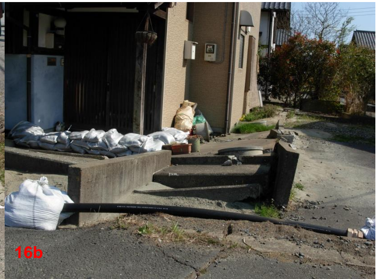
Photo 16a) and 15b). Distortion of the ground in the surrounding area of building. Down of ground level causing severe damage (crack on the sidewalk) and differential settlement on the structure around of the building.
