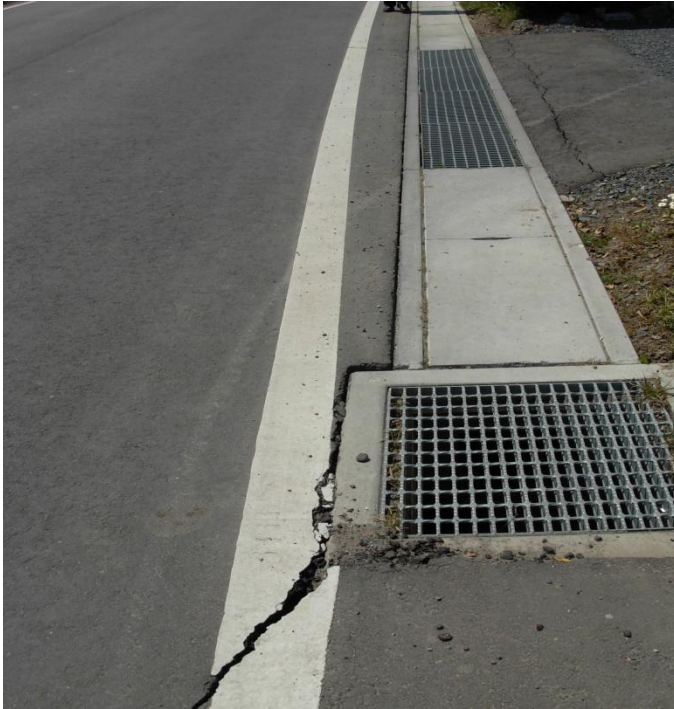
Photo 2. Crack at the border of the road. This kind of damage can be occasioned due lateral displacement not uniform of the ground, because the shaking from the earthquake.
