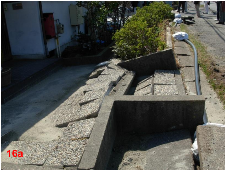
Photo 16a) and 15b). Distortion of the ground in the surrounding area of building. Down of ground level causing severe damage (crack on the sidewalk) and differential settlement on the structure around of the building.
