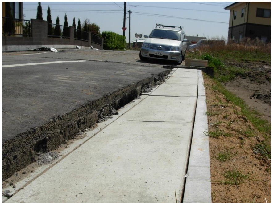
Photo 3. Settlement of the sidewalk. Difference of level, due to liquefaction phenomenon. In this case the settlement of the sidewalk was around 16 cm. This kind of damage is common in area with soil condition susceptible to liquefaction. At this site was possible to observe the liquefaction phenomenon, so, is sure about the cause of this kind of damage.
