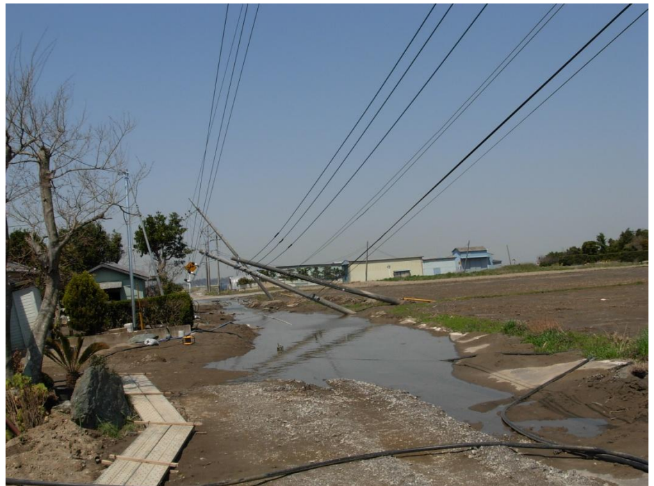
Photo 5. Inclination and collapse of electric post.
