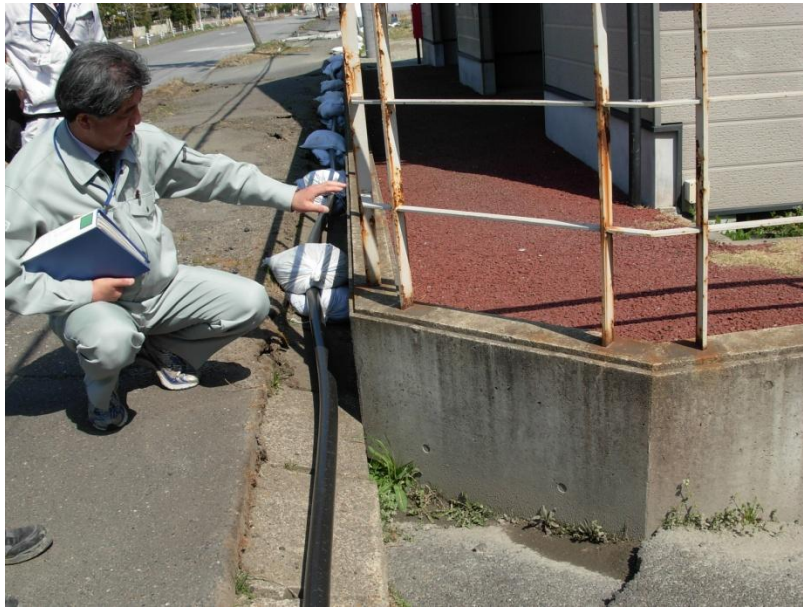
Photo 19. Crack and difference level at the retaining wall. In this case was difficult see, if this wall has steel reinforce, because the crack is not perpendicular to the longitudinal section. On the top of the wall the wide of the crack is around 1.5 cm.
