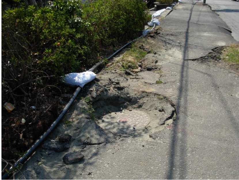
Photo 14. The pipe water went up. After the earthquake the water service remained out of service, this kind of damage is due to liquefaction also.
