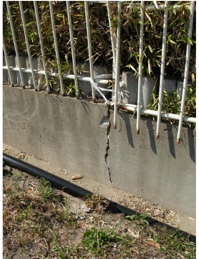
Photo 19. Crack and difference level at the retaining wall. In this case was difficult see, if this wall has steel reinforce, because the crack is not perpendicular to the longitudinal section. On the top of the wall the wide of the crack is around 1.5 cm.
