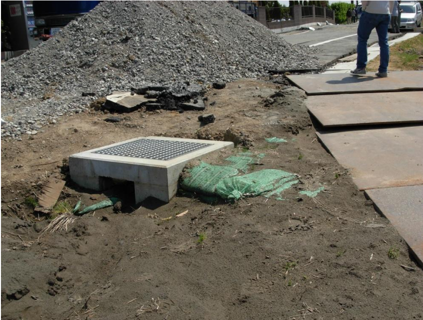
Photo 4. Uplift of the drainage structure. Due to liquefaction phenomenon the structure of the concrete utilized for drainage system was uplifted around 15cm from the original level.
