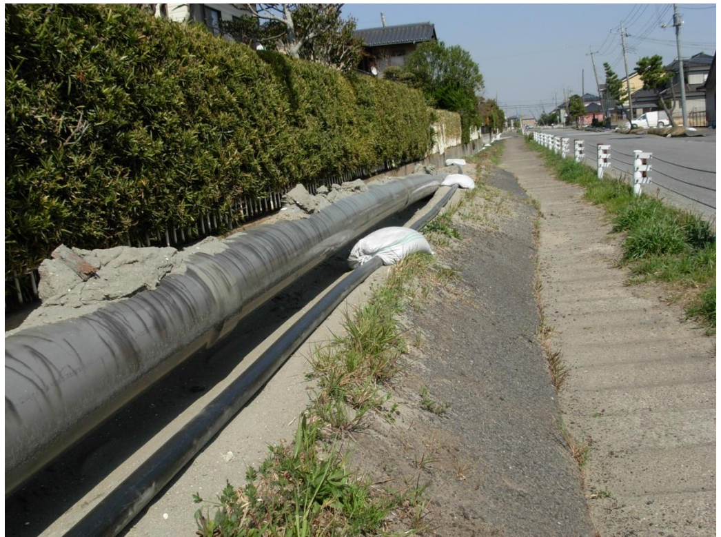
Photo 14. The pipe water went up. After the earthquake the water service remained out of service, this kind of damage is due to liquefaction also.
