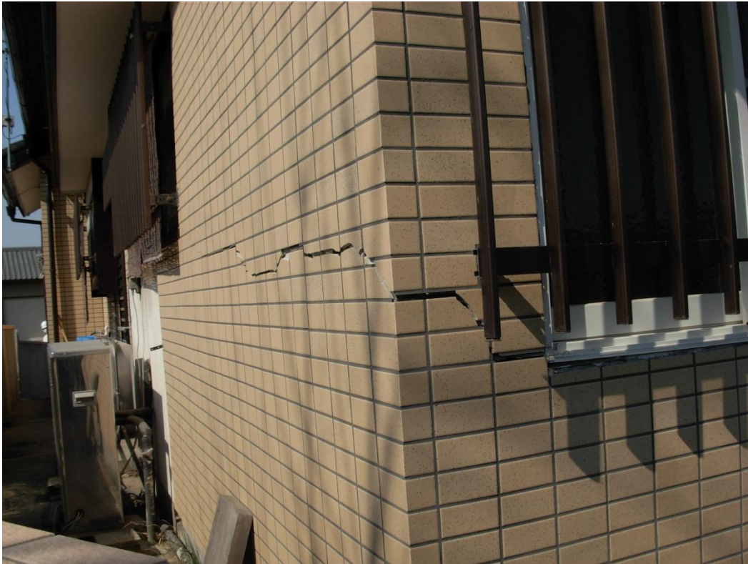
Photo 23. Crack at the house's corner. Due to lateral displacement and settlement in the front side, this house suffered damage in the back side, specifically crack at the both mainly corner.
