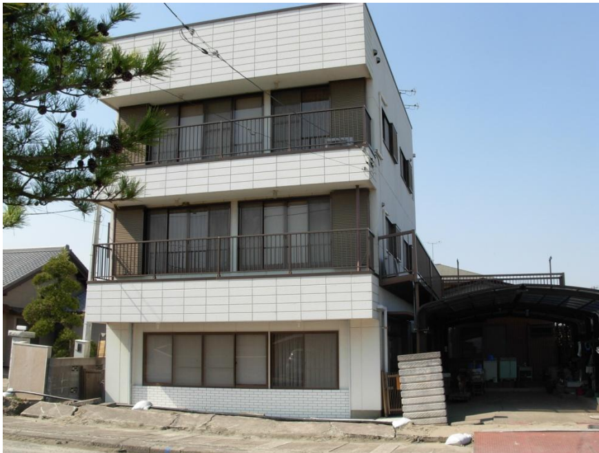
Photo 17. Settlement around of the building. Some case differential settlement can cause the total collapse of the building, however when the settlement is uniform, the building can keep straight, in this case the photo shown good behavior of the building against differential settlement, due that the structure around the building suffered settlement with different magnitude, maybe due to kind of foundation .
