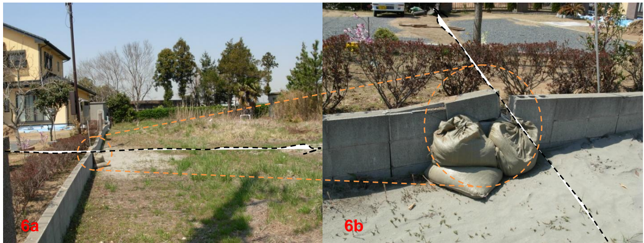
Photo 6a) and 6b). Crack and displacement (vertical and horizontal) in the fence retaining wall (concrete block). Damage due to liquefaction phenomenon, the dash line show the direction of the crack on the ground, the fine sand is evidence of liquefaction, the lateral and vertical displacement on the retaining wall is showed (orange dash circle).
