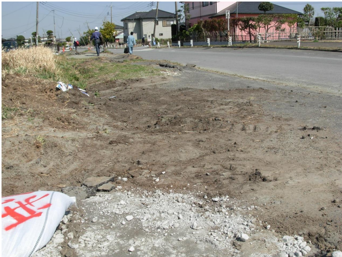
Photo 27. Deformation of the surface ground. Difference of level of the ground, due to settlement occurred.
