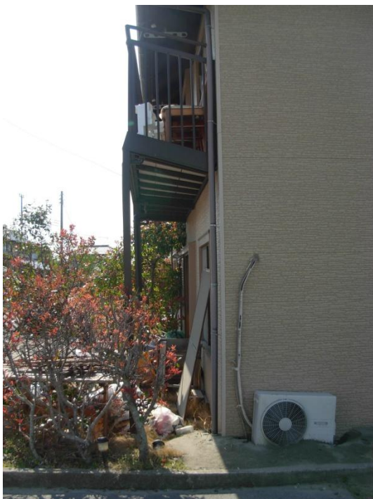
Photo 24. Differential settlement of the two stories building. This kind of damage was observed in several houses around the area visited, this is due to liquefaction phenomenon and foundation condition.
