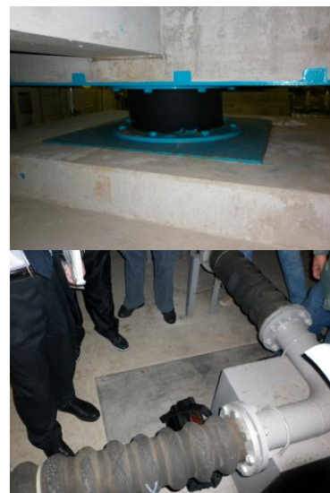
Figure 4. Base isolation system of Suisen-no-ie
