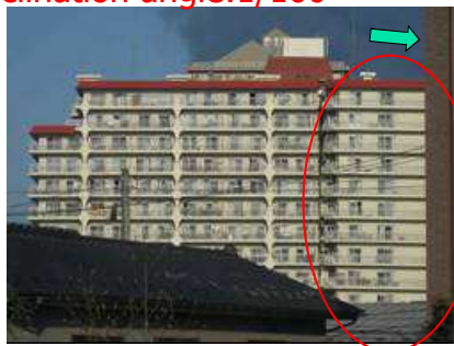
Inclined 14 story SRC building
