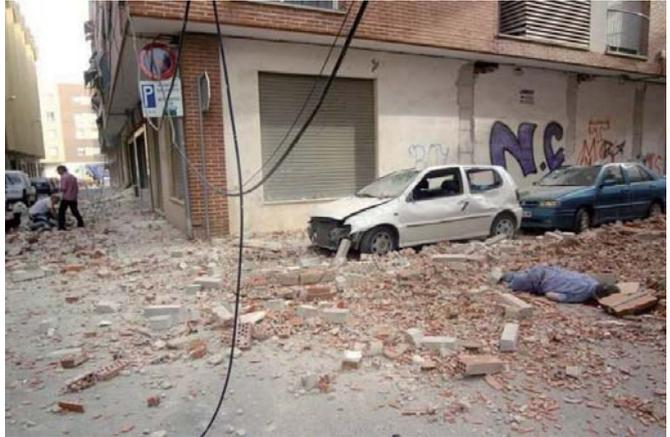
The victims were due to detachments nonstructural elements (sills, parapets, etc.)
