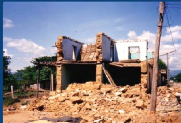
Damage to Tapial construction (1990 Peru EQ)
