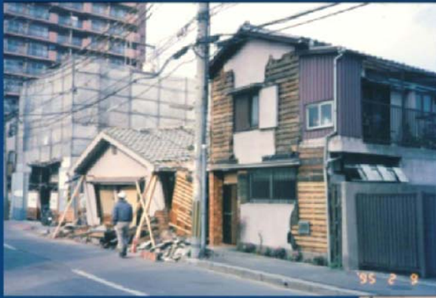
Damage to Japanese traditional wooden houses (1995 Kobe EQ)
