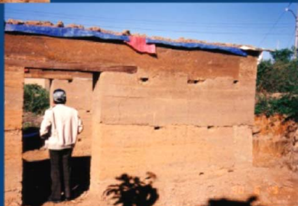
Tapial is cast-in-place mud (rammed earth ) construction (1990 Peru EQ)
