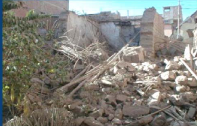
Damage to Adobe (2001 Atico, Peru EQ)
