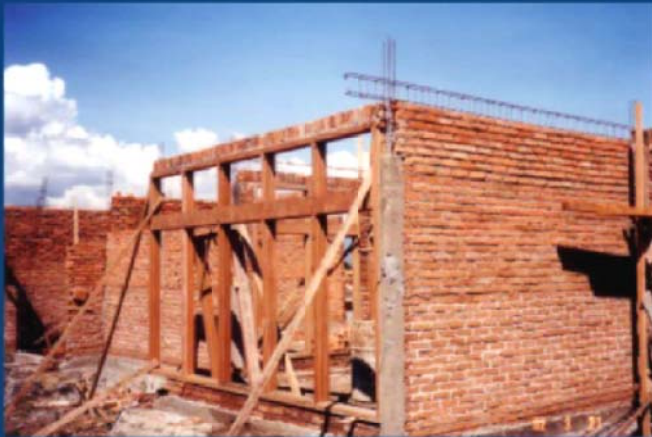
Confined masonry Un-reinforced brick wall farmed with RC columns and beams
