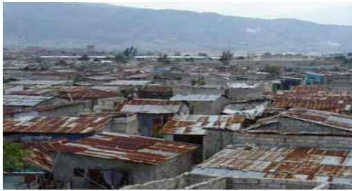
Substandard housing (RES1)
