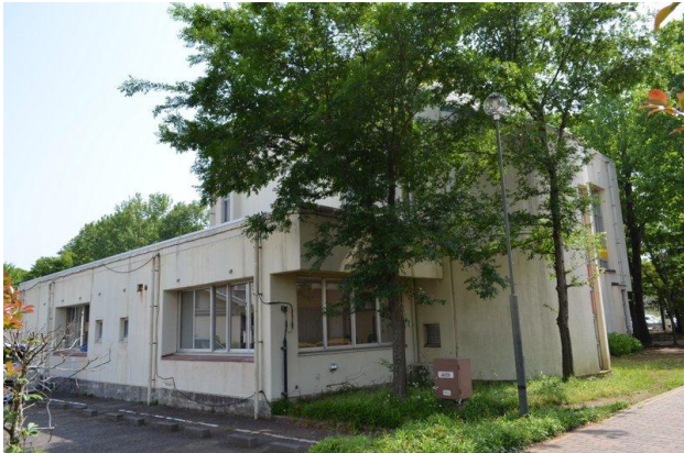
Photo 1. The community center building
