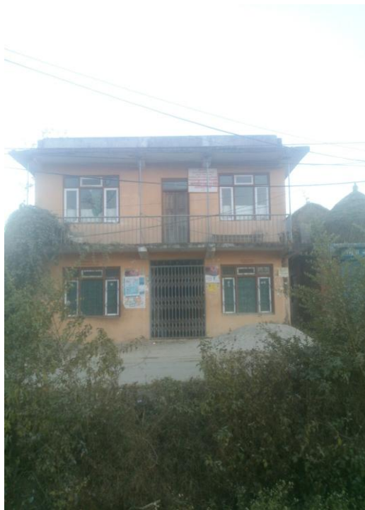
Figure 1. Alapot Health Post Building
