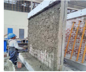
Figure 3. Coatings of steel mesh with mortar.
