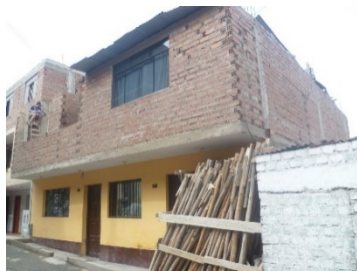
Figure 1. Typical masonry housing in the surroundings of the city of Lima.
