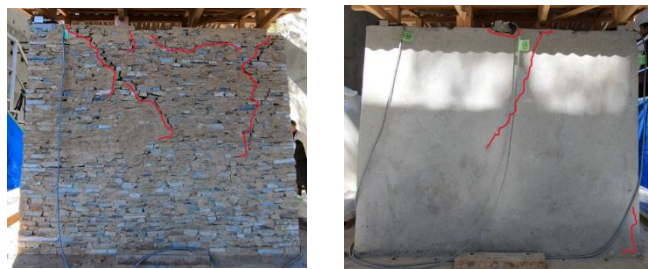
Figure 9. Stone masonry (USM & RSM)
