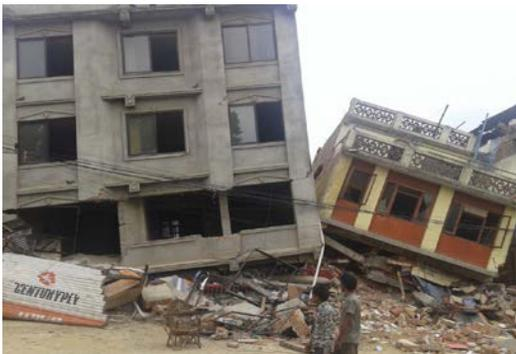
Fig. 1. The soft first stories collapsed in 2015 Gorkha Earthquake Nepal.
